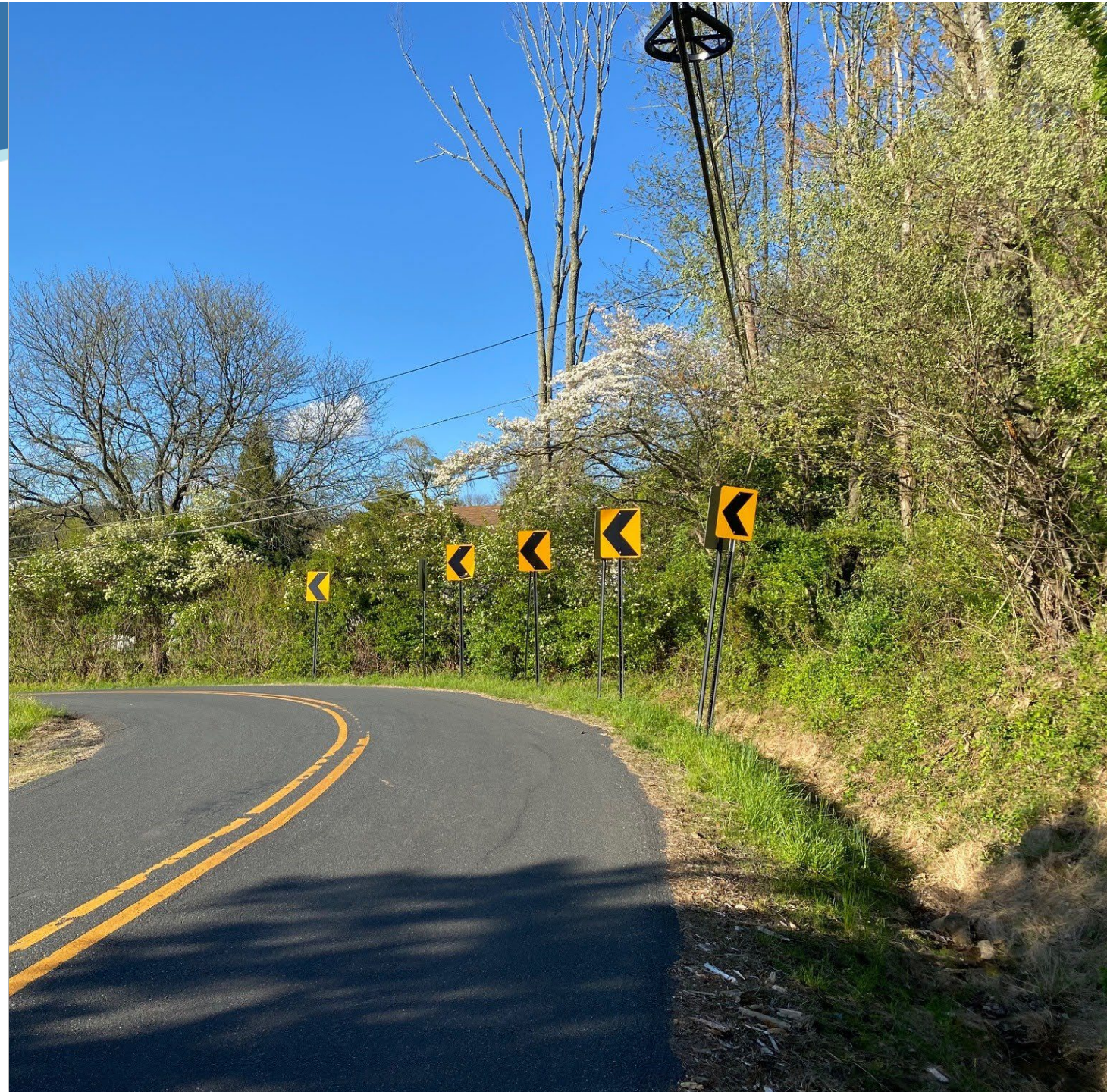
Chevron signs with retroreflective strips on sign posts installed along a curve. Source: FHWA
