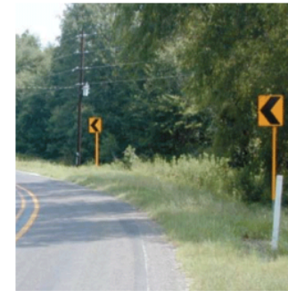
Chevron signs with retroreflective strips on sign posts installed along a curve. Source: FHWA
