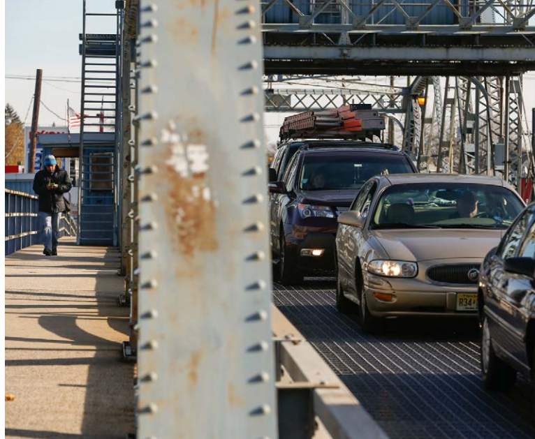
Kingsland Avenue Bridge, Bergen/Essex Counties
