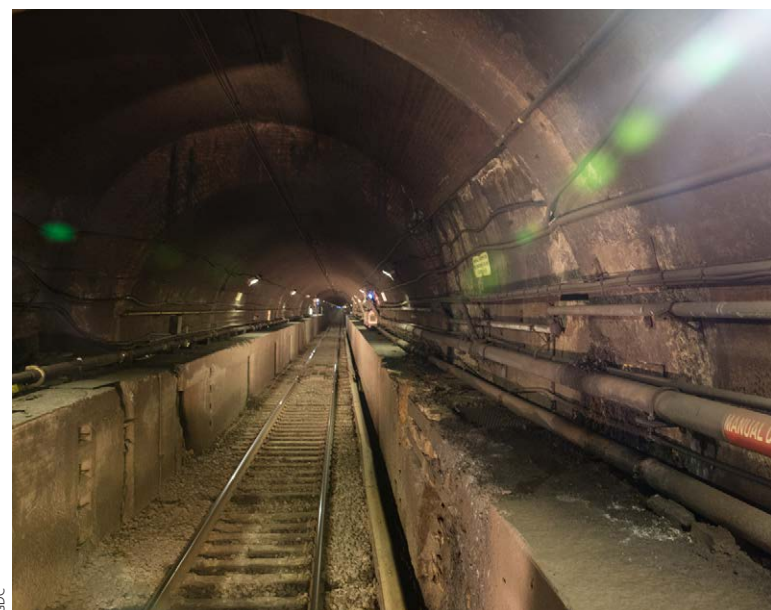
North River Tunnel, Hudson County
