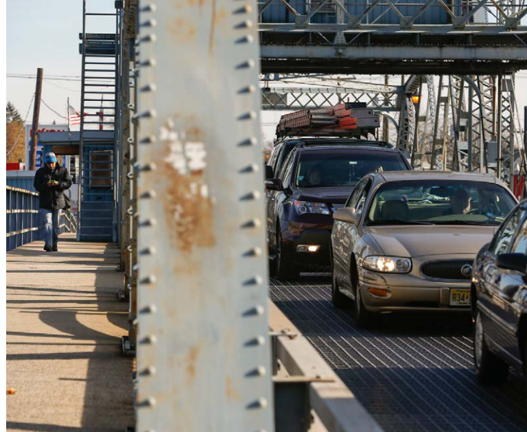
Kingsland Avenue Bridge, Bergen/Essex Counties
