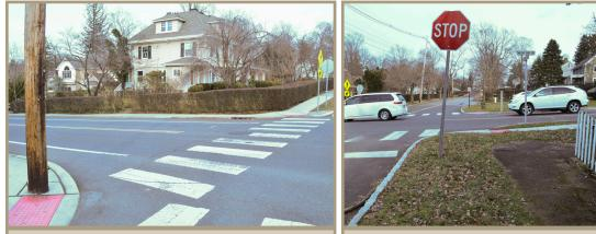
Figure 37. High visibility crosswalks, ADA compliant ramps, and pedestrian signage at Mt. Airy Road.
