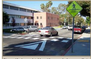
Figure 45. A speed table with a marked crosswalk (a raised crosswalk).
