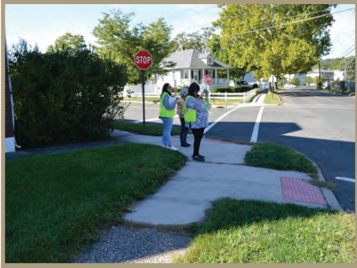
Figure 17. ADA-compliant curb ramps,
