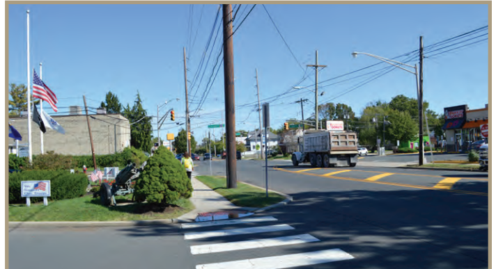
Figure 37. Looking south across Union Avenue. There is no crosswalk for pedestrians or bicyclists.
