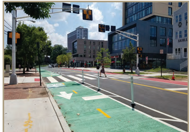
Figure 3. This Complete Street in New Brunswick, NJ, features a bicycle path, bus lane, and enhanced pedestrian crossing.
