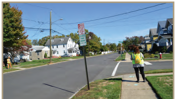
Figure 24. Intersection of Maple Avenue and Clearview Place. Parking signage does not advise drivers against parking too close to the corner. There is no crosswalk across Maple.
