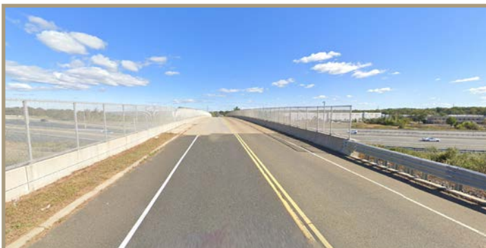
Figure 46. Half Acre Road over the NJ Turnpike.
