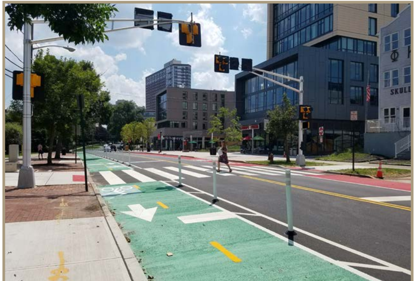
Figure 3. A complete street, as seen in New Brunswick, New Jersey. No two complete streets are alike, as they should always reflect the context of the street and the character of the community.
