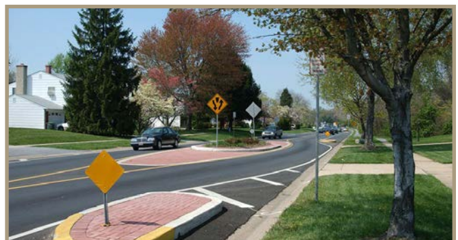
Figure 21. A median island used for traffic calming. (Source: NACTO)
