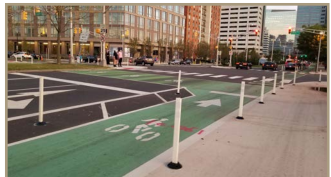
Figure 69. A painted curb extension and bicycle box in Jersey City, NJ.
