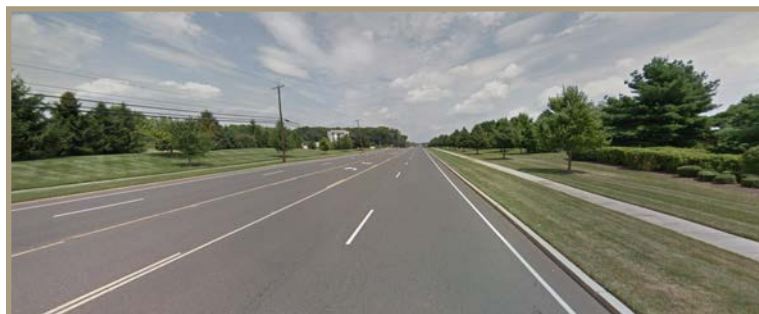
Figure 72. Looking north on South River Road, past Liberty Dr.
