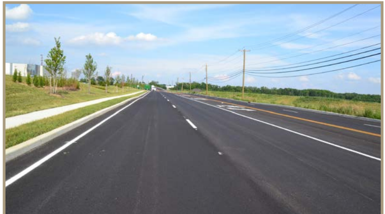
Figure 39. Looking east along the newly widened section of Half Acre Road. The new warehouse complex is on the left.
