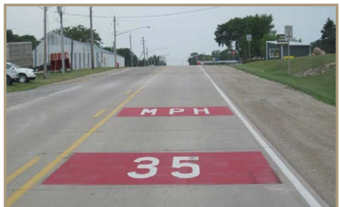
Figure 19. Speed limits may be reinforced with pavement markings, as seen in Slater, Iowa.. (Source: FHWA)
