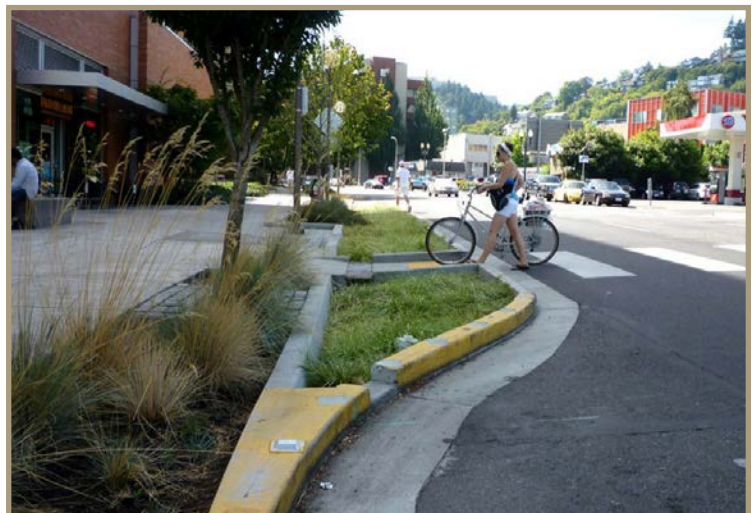
Figure 10. Green infrastructure used to narrow the roadway and provide a shorter crossing distance for pedestrians.
