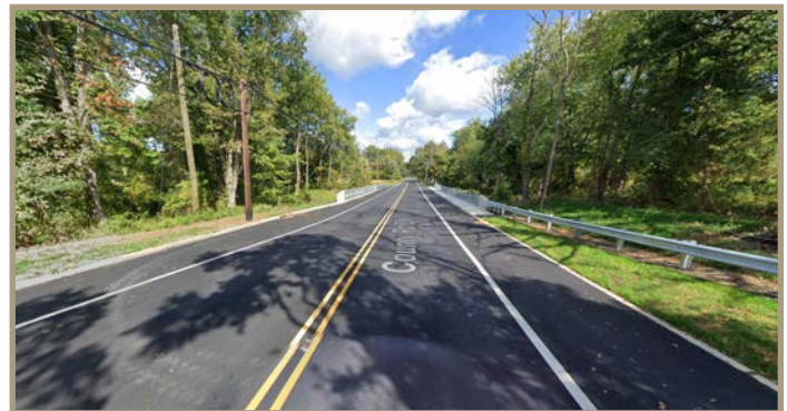
Figure 49. Looking north on Main Street to the newly widened bridge.
