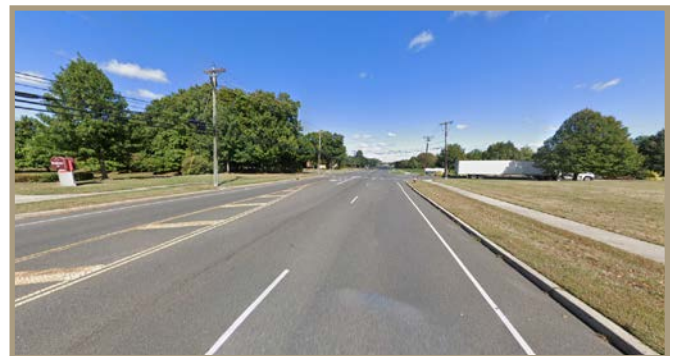
Figure 71. Looking north on South River Rd., prior to Security Dr.
