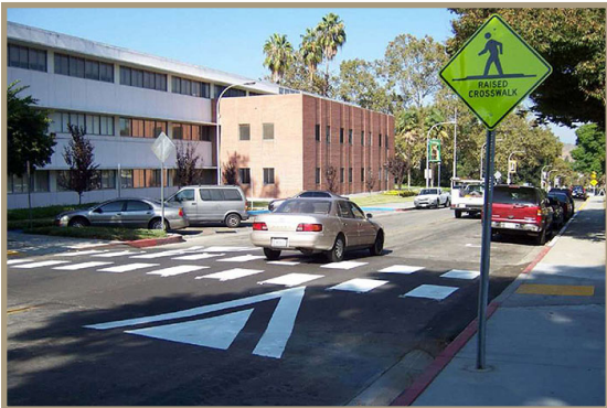
Figure 51. A speed table with a marked crosswalk (a raised crosswalk).
