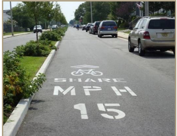
Figure 50. Pavement markings in Ocean City, New Jersey.
