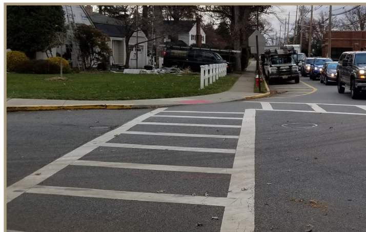
Figure 44. It is best practice to build a ramp oriented directly into each crosswalk, rather than a single diagonal ramp shown here.
