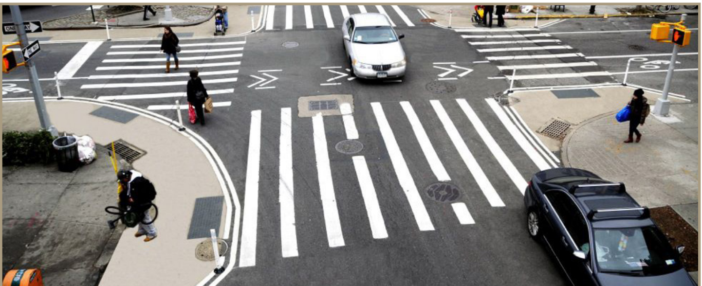
Figure 60. New York City has made extensive use of paint and plastic bollards to decrease turn radii at intersections throughout the city.
