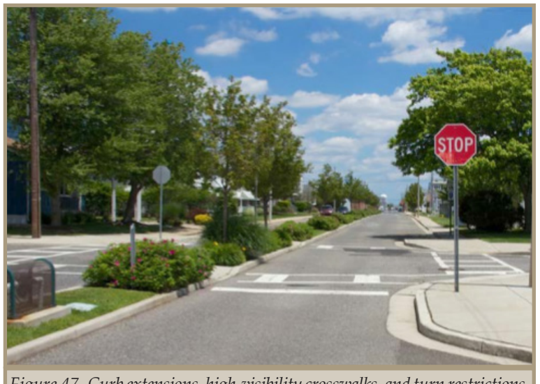
Figure 47. Curb extensions, high-visibility crosswalks, and turn restrictions calm traffic along a bicycle boulevard in Ocean City, NJ.
