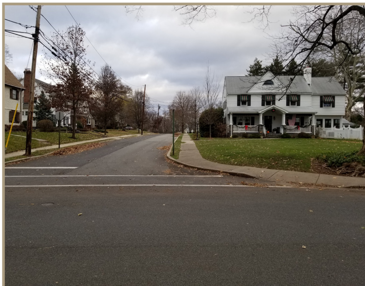
Figure 20. Wide turn radius at various intersections.
