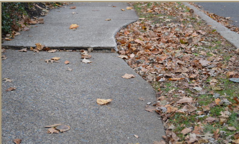
Figure 14. The sidewalk frequently narrows where mature trees once stood. The roots of those trees have raised the sidewalks at some locations.
