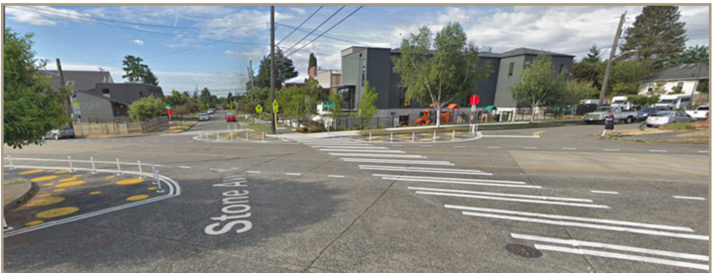
Figure 57. Curb extensions using plastic bollards and paint have been used in Seattle to realign confusing intersections, slow traffic, and add new pedestrian crossings.
