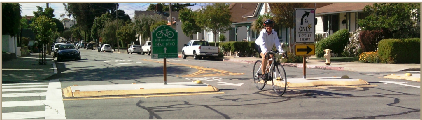
Figure 53. Diverters in San Luis Obispo, California, force automobile traffic to turn, while allowing bicyclists to continue straight.
