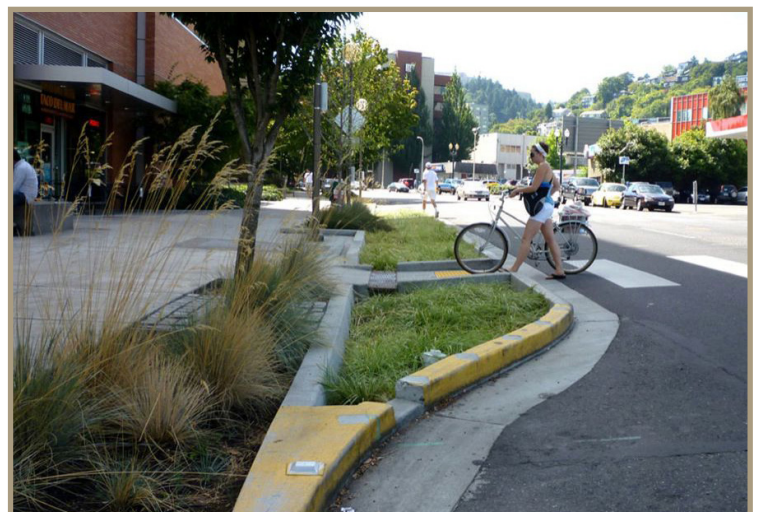
Figure 55. Green infrastructure used to narrow the roadway and provide a shorter crossing distance for pedestrians.
