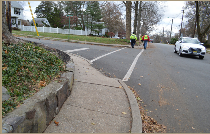
Figure 38. At Gramercy Place, the sidewalk narrows, there is a strong cross-slope, the corner ramp is not ADA compliant, and the wide turning radius encourages faster vehicle speeds.
