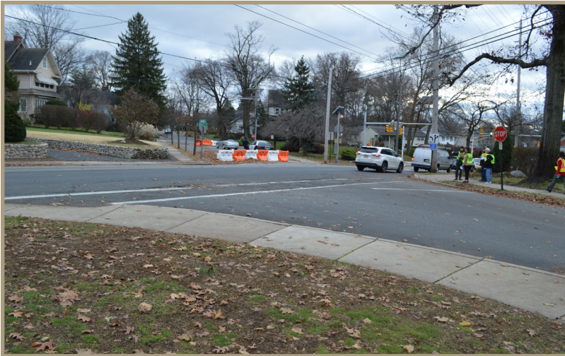
Figure 30. Very wide turning radius at the intersection of Hamilton and Maple.
