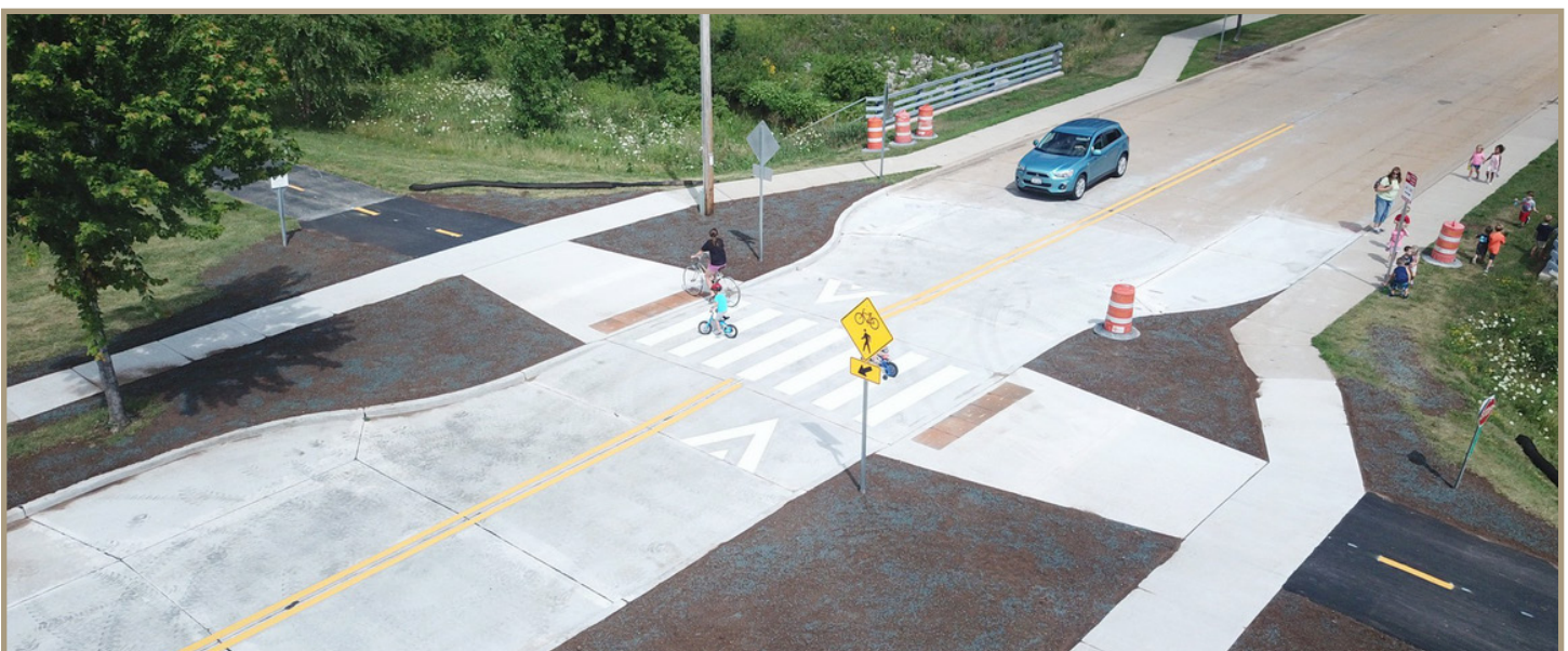
Figure 65. A raised crosswalk at a trail crossing in Appleton, WI.
