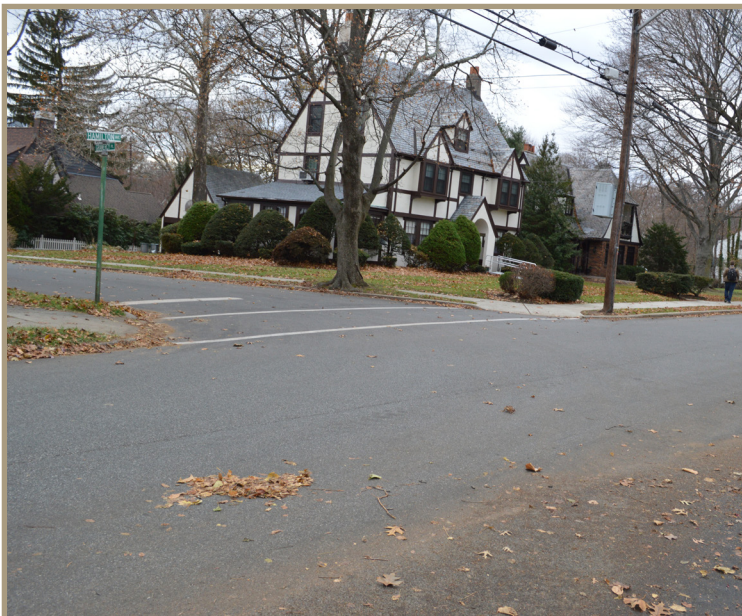
Figure 18. Crosswalks across Hamilton Avenue are absent at the various T-intersections, (looking north on Hamilton Avenue).
