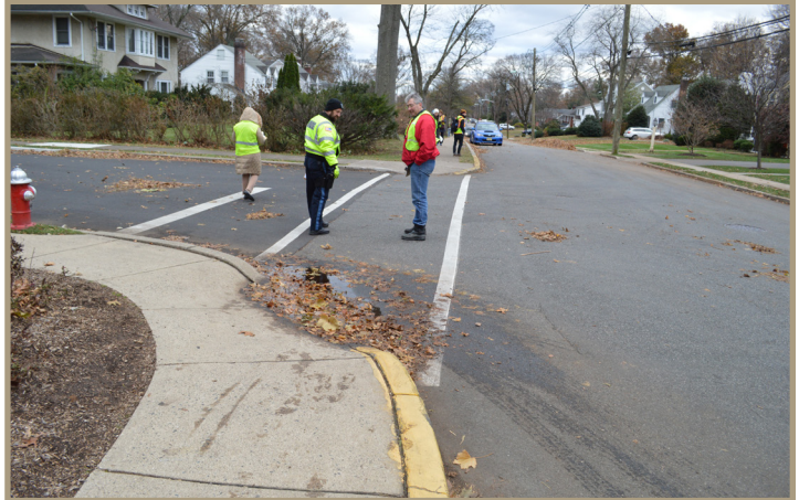
Figure 39. The curb ramp at Emerson Road accumulates debris, and is not ADA compliant. There is no marked crosswalk across Hamilton Avenue.
