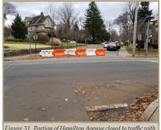
Figure 31. Portion of Hamilton Avenue closed to traffic with temporary traffic control.
