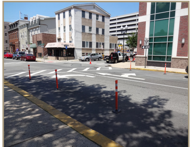
Figure 56. New Brunswick, NJ, uses plastic bollards to prevent illegal parking near intersections. After a successful trial at one intersection, the city has added them throughout the city.
