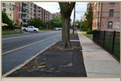
Figure 43. Crumbling pavement between the sidewalk and travel lane.
