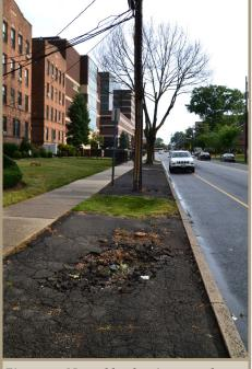
Figure 16. Unusable planting area due to unmaintained pavement.
