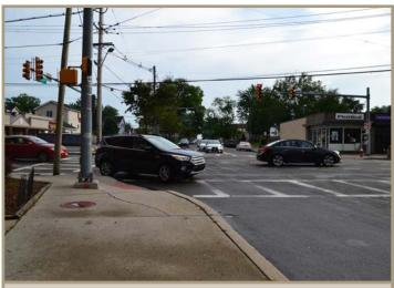
Figure 32. Looking south on Prospect Ave. toward Essex St. The curb ramps are not ADA compliant and the sidewalk narrows due to the traffic signal.
