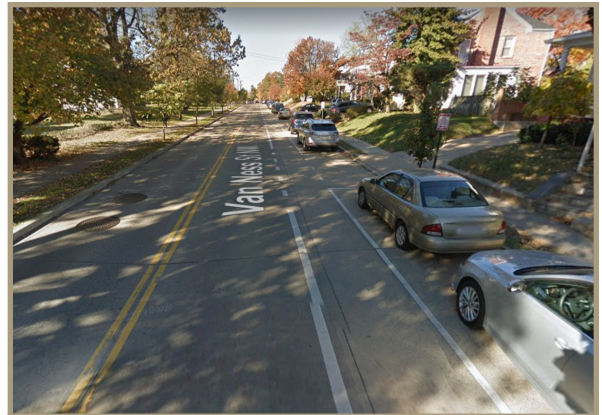
Figure 35. A climbing bicycle lane on Van Ness Street NW, in Washington D.C.
