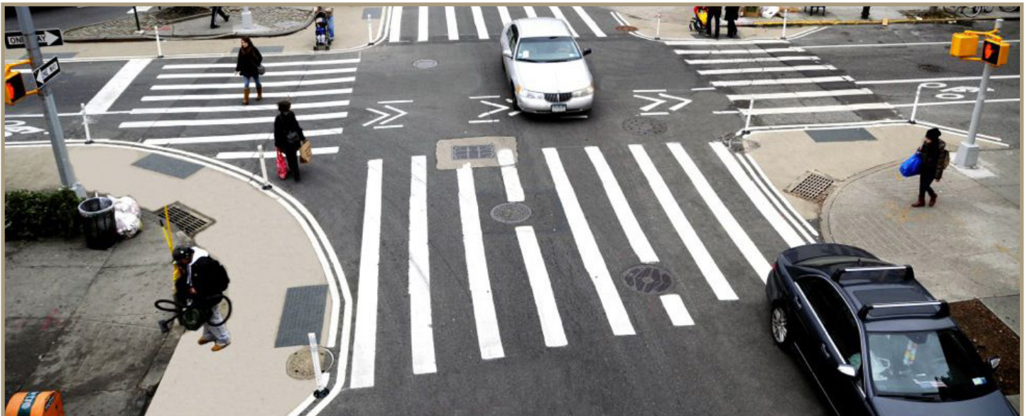
Figure 58. New York City has made extensive use of paint and plastic bollards to decrease turn radii at intersections throughout the city.
