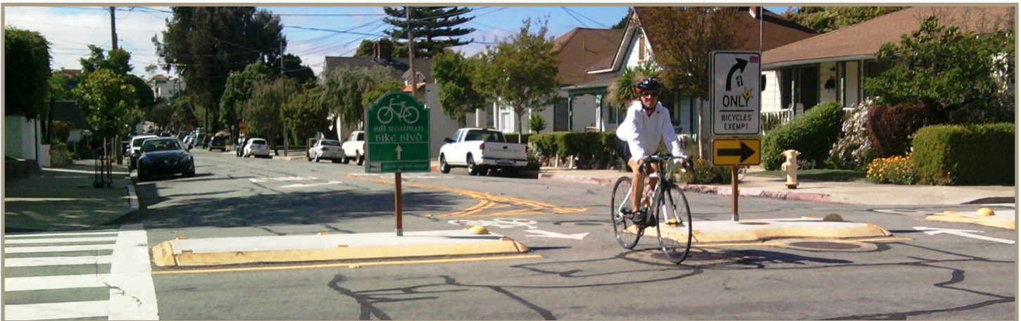
Figure 51. Diverters in San Luis Obispo, California, force automobile traffic to turn, while allowing bicyclists to continue straight.
