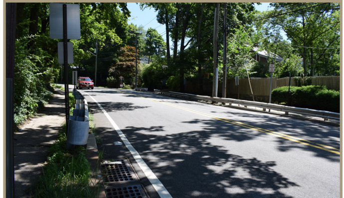
Figure 32. Looking southeast on Fort Lee Road, at Glenwood Avenue.
