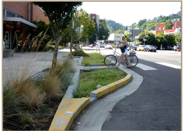
Figure 53. Green infrastructure used to narrow the roadway and provide a shorter crossing distance for pedestrians.
