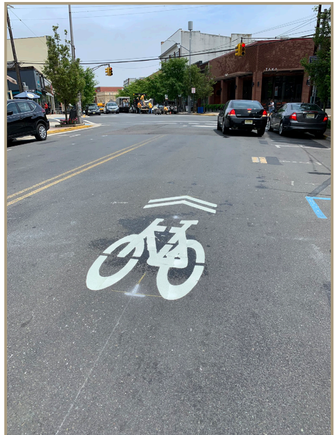
Figure 59. Sharrow installed in Asbury Park in May 2019, as part of their bicycle master plan implementation process.
