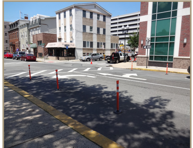
Figure 54. New Brunswick, NJ, uses plastic bollards to prevent illegal parking near intersections. After a successful trial at one intersection, the city has added them throughout the city.
