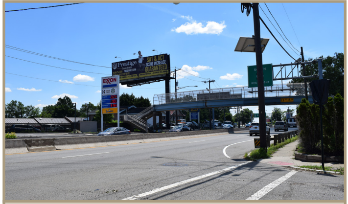
Figure 40. Pedestrian bridge across North Bergen Boulevard, looking south.
