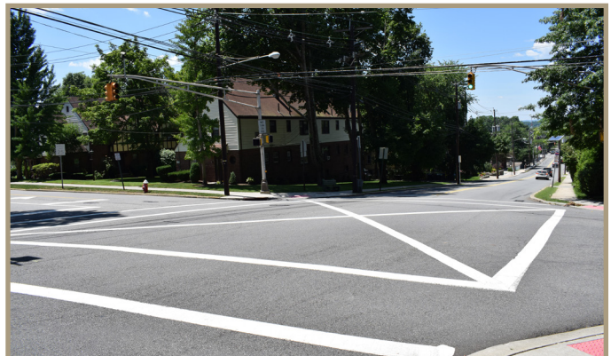
Figure 33. Looking northwest on Fort Lee Road, at Glenwood Avenue.
