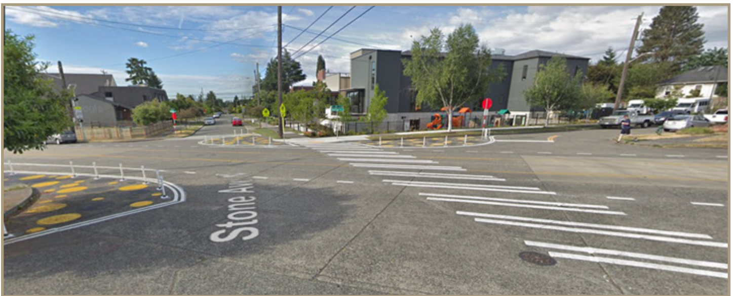
Figure 55. Curb extensions using plastic bollards and paint have been used in Seattle to realign confusing intersections, slow traffic, and add new pedestrian crossings.
