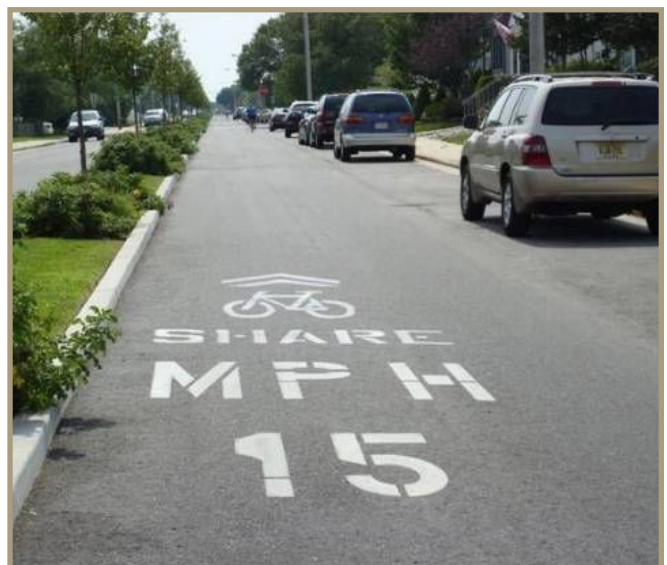
Figure 33. Pavement markings for a bicycle boulevard in Ocean City, New Jersey.
