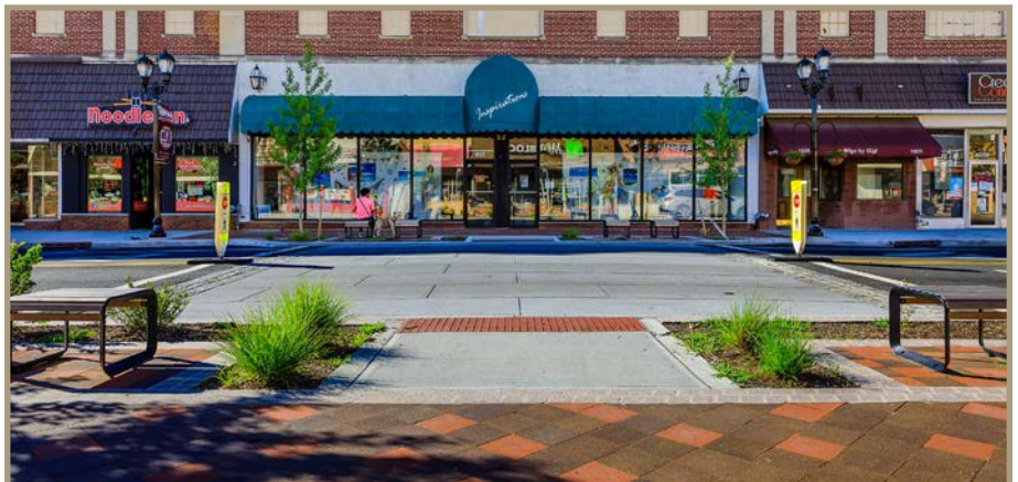
Figure 23. Example of a raised crosswalk in Union, NJ.
