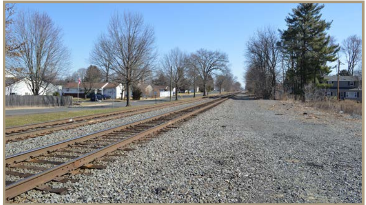
Figure 50. The railroad is at grade level, facilitating the installation of a second grade crossing.
