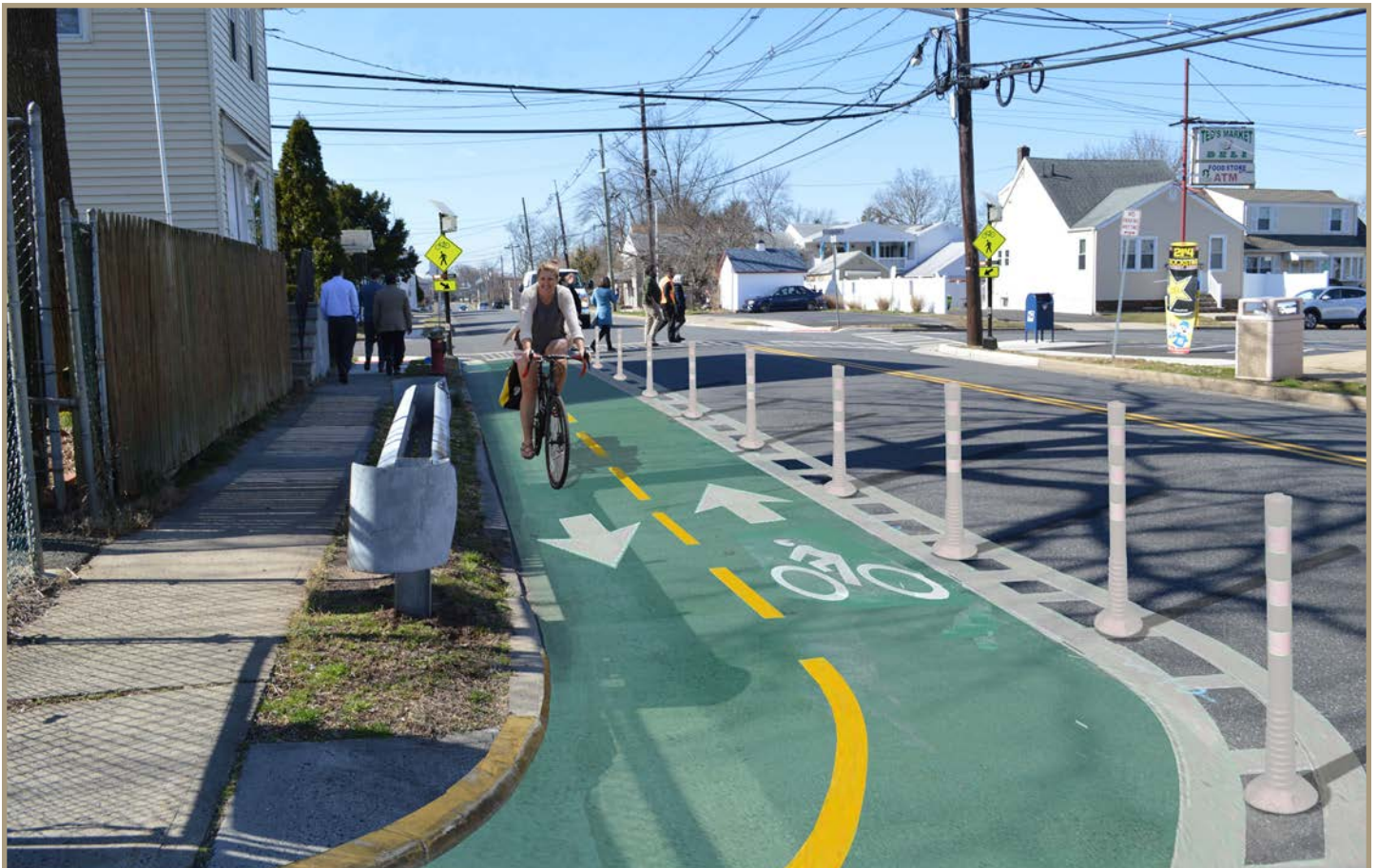
Figure 29. Photo simulation of proposed on-road bicycle path on Kennedy Boulevard, looking south. The flexible plastic bollards may be substituted for a solid barrier for improved safety to bicyclists. However, access to an existing fire hydrant must be maintained.
