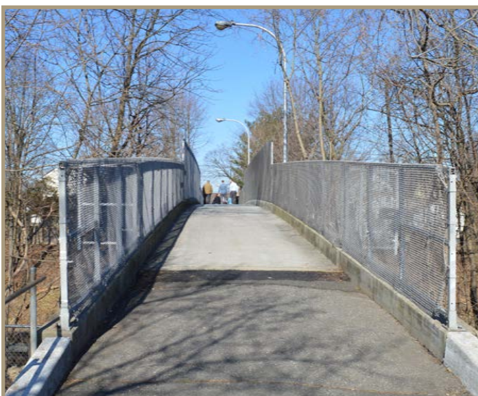
Figure 19. The bicycle and pedestrian bridge over the railroad.
