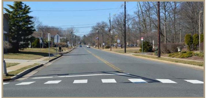
Figure 67. Looking west on Brooks Boulevard, from 13th Avenue.
