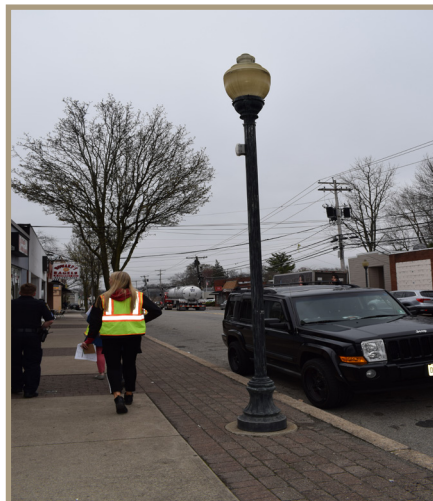
Figure 23. Pedestrian lighting that does not direct light onto the sidewalk, looking southward on North Beverwyck Road near the intersection of Hiawatha Boulevard.
