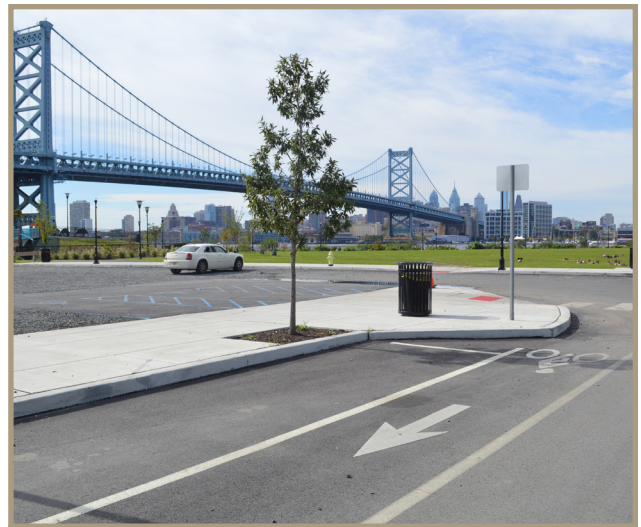
Figure 46. A curb extension in Camden, New Jersey shortens the crosswalk distance and increases pedestrian visibility.
