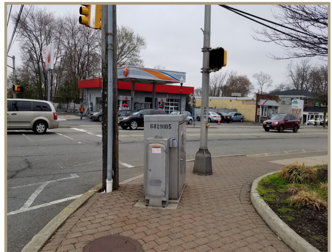
Figure 30. Access to the only ramp located at the southwest corner of the Lake Shore Drive intersection is constricted by the placement of a traffic signal controller box, pedestrian signal, and telephone pole.
