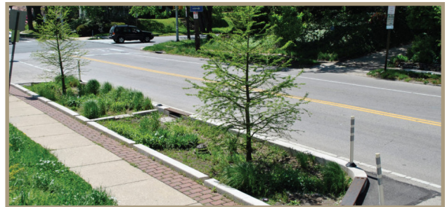
Figure 38. Green infrastructure used to narrow the roadway in Philadelphia, PA, also creates a buffer between pedestrians and passing traffic and can be used on curb extensions that shorten the crosswalk distance.
