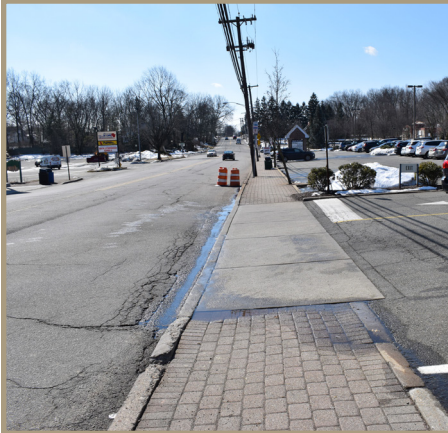
Figure 33. Wide storefront driveway with sloping sidewalks, looking southward on North Beverwyck Road near Claudine Terrace.
