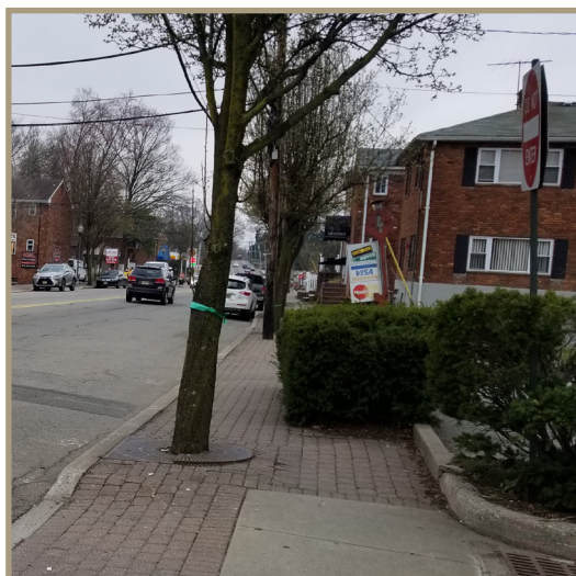
Figure 31. Cluttered sidewalks with uneven pavers, tree well grates, and overgrown bushes, looking south on North Beverwyck Road.
