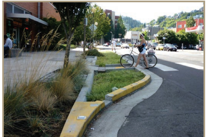
Figure 6. Green infrastructure used to narrow the roadway and provide a shorter crossing distance for pedestrians.
