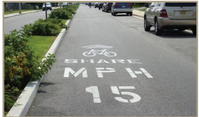
Figure 17. Pavement markings for a bicycle boulevard in Ocean City, New Jersey.
