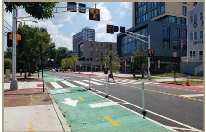
Figure 3. This Complete Street in New Brunswick, NJ, features a bicycle path, bus lane, and enhanced pedestrian crossing.
