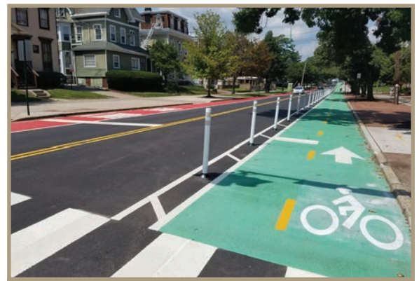
Figure 34. Two-way bicycle lane in New Brunswick, NJ.
