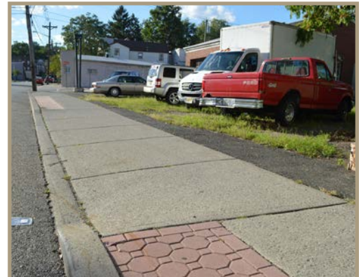
Figure 48. Driveway north of Watson Avenue.
