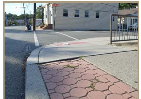
Figure 19. Tripping hazard at end of furnishing zone.
