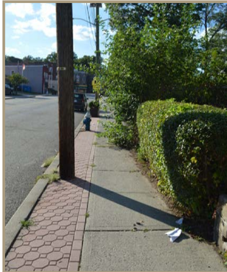
Figure 16. Looking north on Washington Street, a narrow sidewalk is limited by overgrown bushes on a neighboring property.
