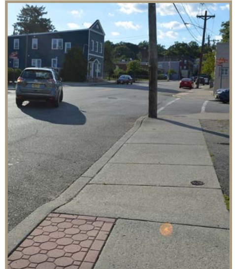
Figure 17. Looking north on Washington Street, a driveway creates a cross slope along the sidewalk.
