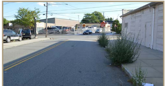
Figure 51. Looking south on Whittlesey Avenue toward Washington Street. Overgrown weeds are visible.
