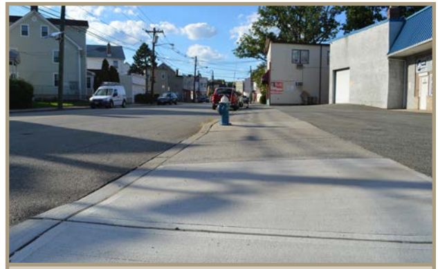
Figure 35. Sloped sidewalk due to commercial driveway.
