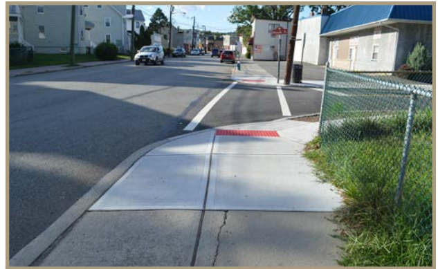
Figure 32. Looking north on Washington Street, to brand new ADA-compliant curb ramps across Meade Street.
