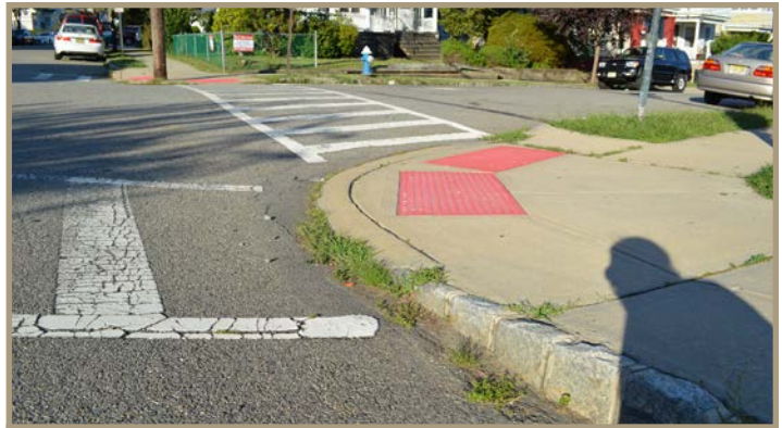
Figure 69. Curb ramps on the corner of Franklin Avenue and William Street.
