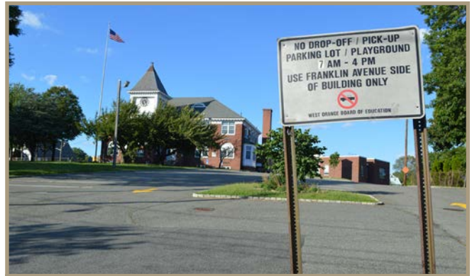
Figure 55. The Washington School parking lot, as seen from Washington Street.
