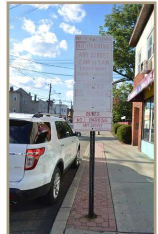
Figure 34. Faded signage on Washington Street.
