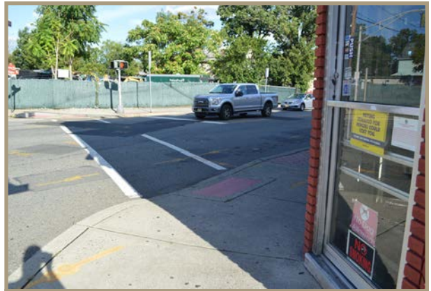
Figure 38. The angle of the intersection creates a tight squeeze for pedestrians on the southwest corner.
