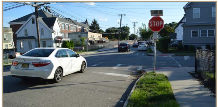
Figure 24. Looking south at Franklin Ave. and William St. Flashing red LEDs activate on the border of the stop sign when vehicles approach. Crosswalks have high-visibility striping, but need a new coat of paint.
