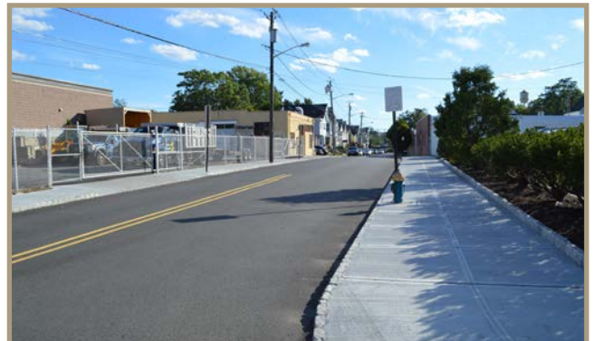
Figure 50. Looking south on Columbia Street, with new sidewalks on both sides.
