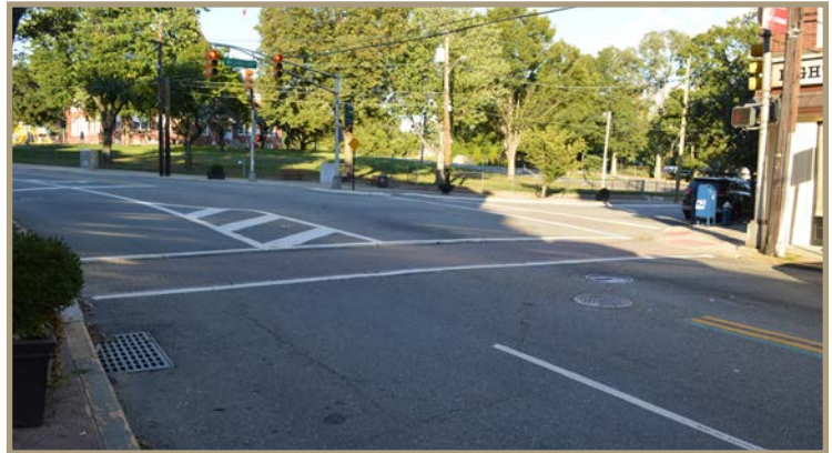
Figure 23. Brick crosswalks at Washington Street and Main Street, looking east.
