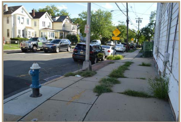
Figure 41. Overgrown sidewalk on Watchung Avenue.
