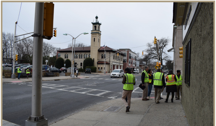
Figure 21. Pedestrian signal heads are missing at the intersection of Elm Street and North Avenue.
