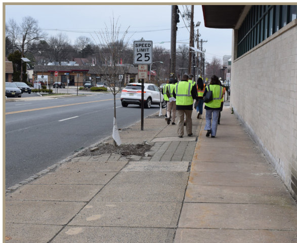
Figure 33. No barrier between pedestrians and large volumes of traffic, looking eastward on North Avenue near Central Avenue.
