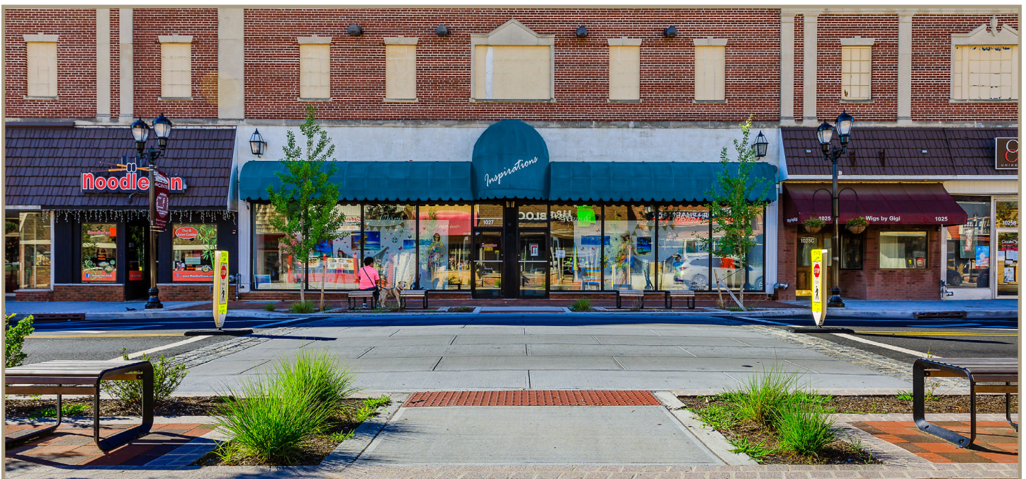
Figure 65. A sidewalk-level midblock crossing on Stuyvesant Avenue in Union Township, New Jersey. (Photo and design courtesy of Arterial LLC)
