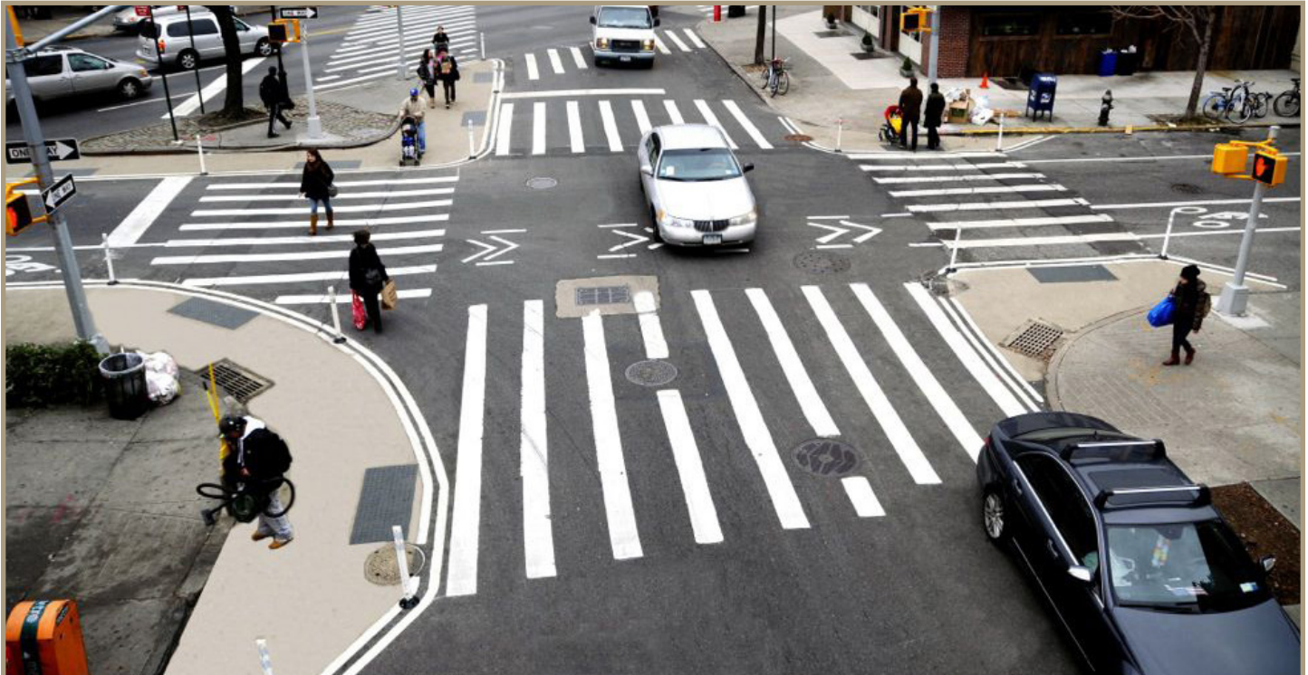
Figure 63. New York City has made extensive use of paint and plastic bollards to decrease turn radii at intersections throughout the city.
