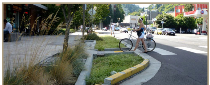
Figure 50. Green infrastructure used to narrow the roadway and provide a shorter crossing distance for pedestrians. (Photo credit: NACTO)
