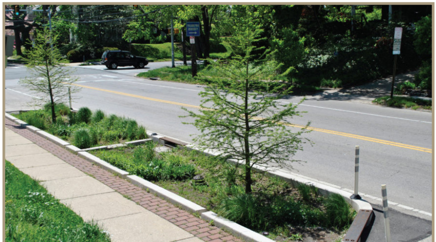
Figure 55. Curb extension with green infrastructure to manage stormwater in Philadelphia, PA. (Photo credit: Philadelphia Water Department)
