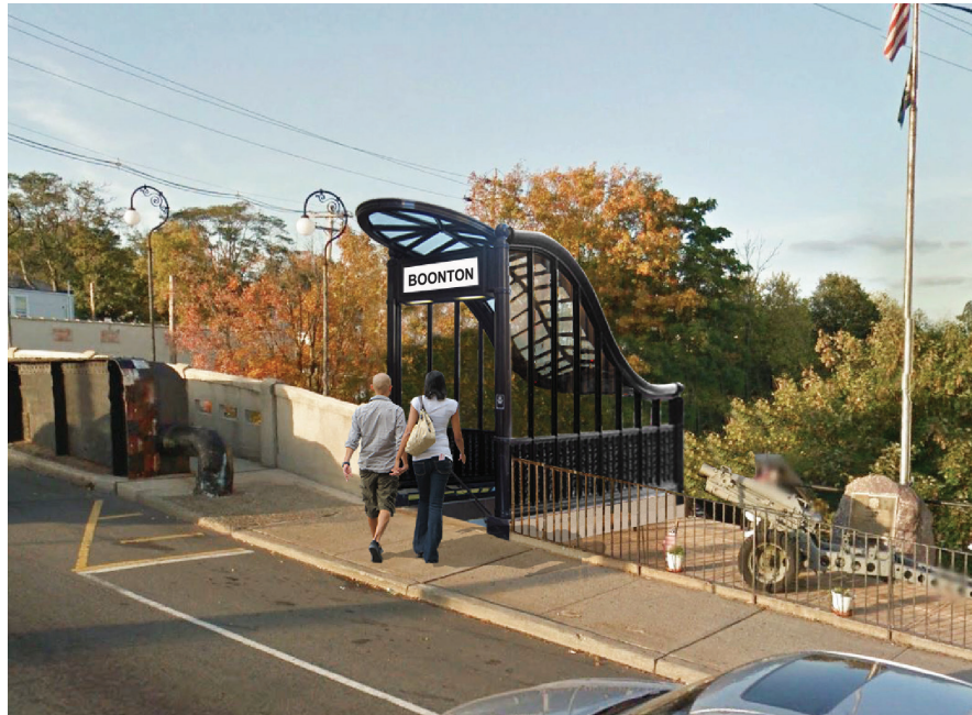
Figure 11: New Staircase to Platform
