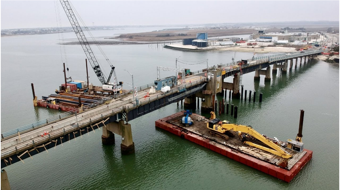
Middle Thorofare Bridge Rehabilitation, 2021 (Source: American Journal of Transportation)
