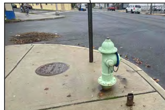
Missing curb ramps and crosswalk, tripping hazard near hydrant
