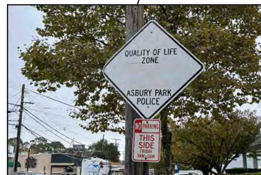
Faded sign, not MUCTD compliant
