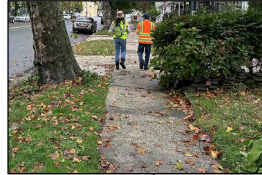
Sidewalk uneven / raised from street trees
