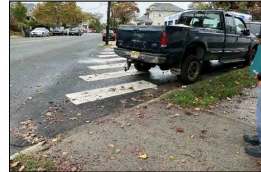
Parked vehicle blocks crosswalk, ramps not ADA compliant
