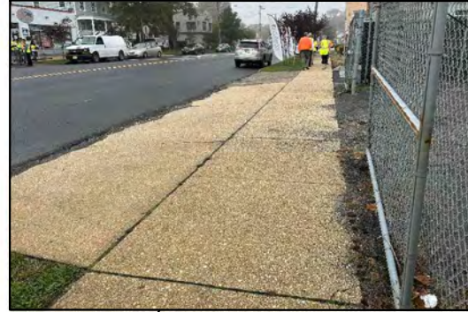
Wide driveway that is not well defined
