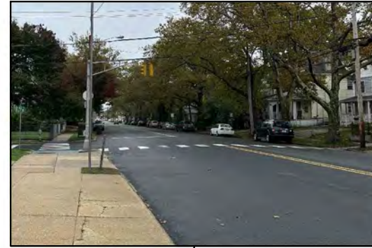
300 feet between stop bars (Pine St to Church St) may be confusing to road users
