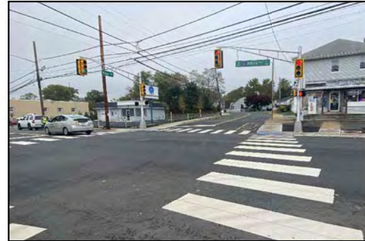
Signal recently upgraded, may need additional intersection lighting
