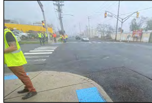
Outdated signal equipment, no pedestrian signal heads, worn crosswalk markings
