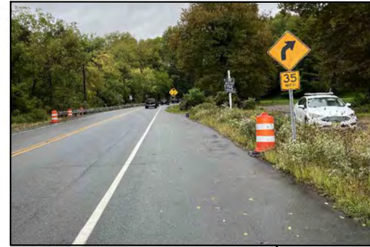
Underpass with low clearance not visible from intersection, shoulders narrow
