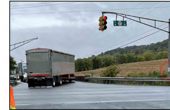
Heavy vehicle turns require stop bars to be farther from intersection, inaccessible push button
