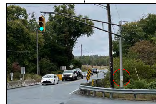
No pedestrian signal heads, push button not accessible behind guide rail
