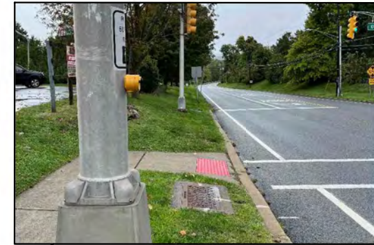
No marked crosswalk or indication to motorists that pedestrians should be expected
