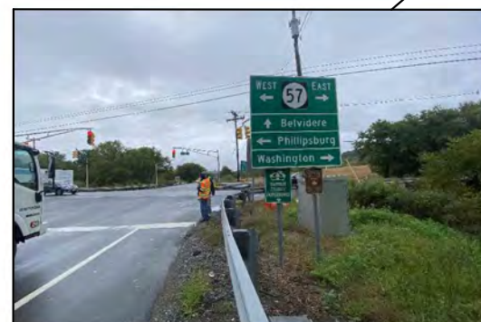
Missing section of sidewalk; no connection for pedestrians between intersections
