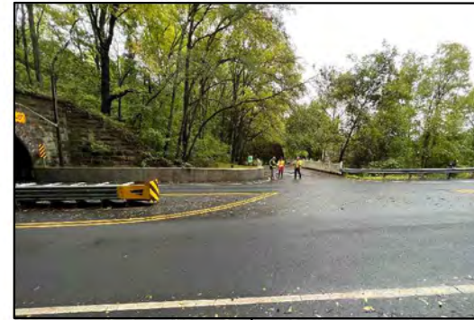
Missing curb ramp; no marked crosswalk
