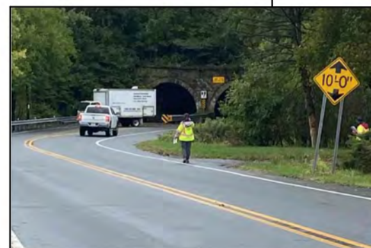
Box truck executing K-turn at underpass due to low clearance and despite warning signs
