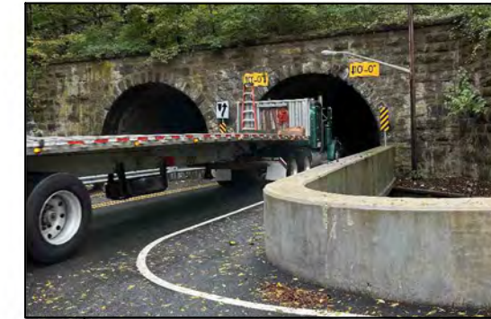
Larger vehicles cannot fit through underpass
