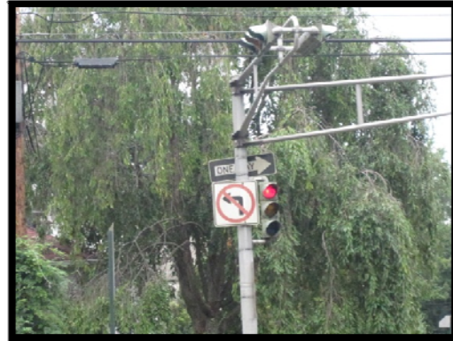
"One Way" sign blocked by pole
