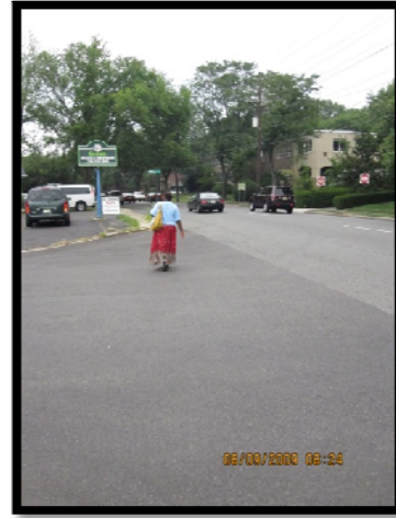
Wide curb radius makes street crossing wider, exposing pedestrians to traffic.
