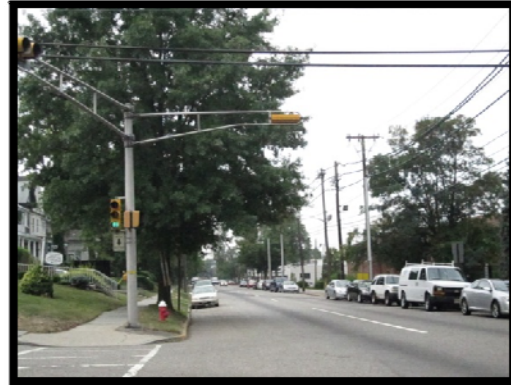
Overhead traffic signal blocked by tree branches
