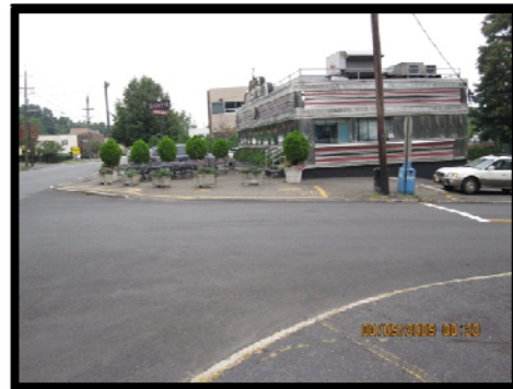
Vehicles stopped at the stop bar are unable to see oncoming traffic.
