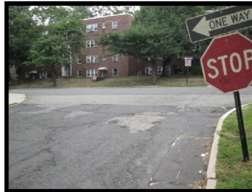
Absence of crosswalk and stop line
