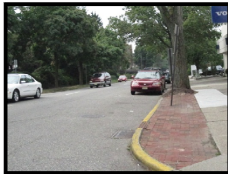
Poor sight distance for vehicles on eastbound approach of Chestnut Street
