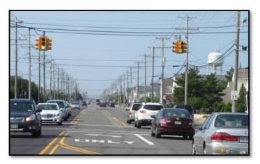
Figure 3a – Horizontal signal on span wire
