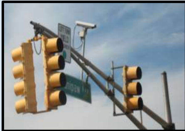
Red light cameras were installed on JFK Boulevard in 2011 and quite likely account for the increase in rear-ended crashes.
