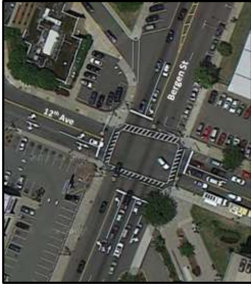
Figure 4 – 12 th Avenue and Bergen Street
