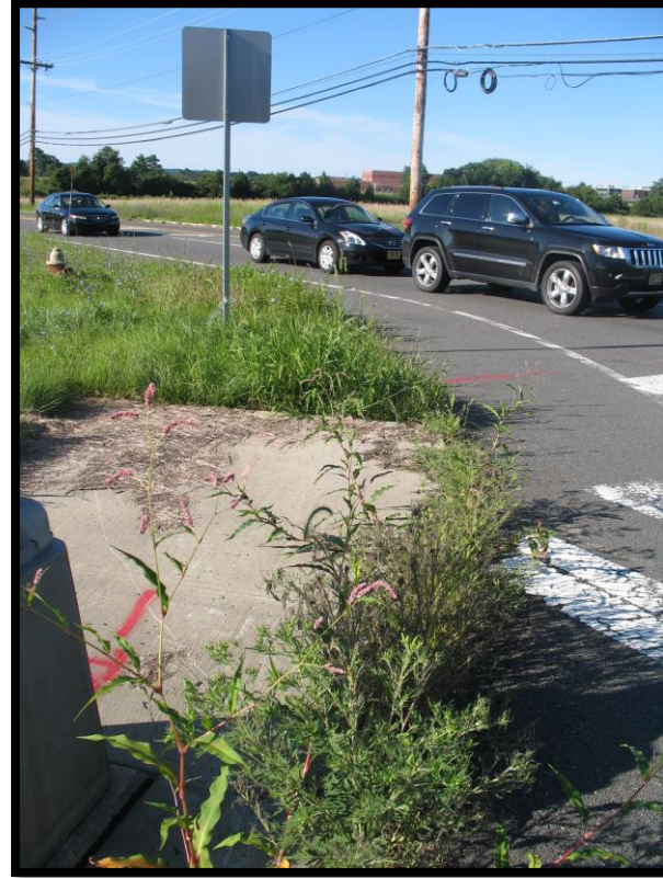
Condition of ramp in southeast corner
