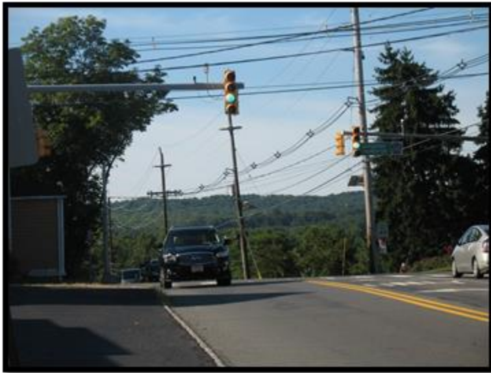
Vertical curve limits sight distance
