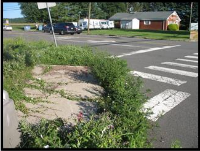
Condition of ramps at northeast corner
