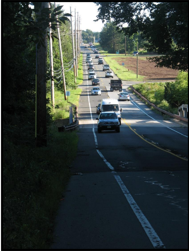
Varying shoulder width is insufficient for bicycles and pedestrians
