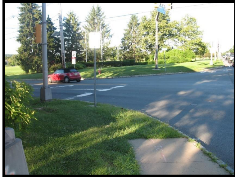
ADA facilities are not compliant
