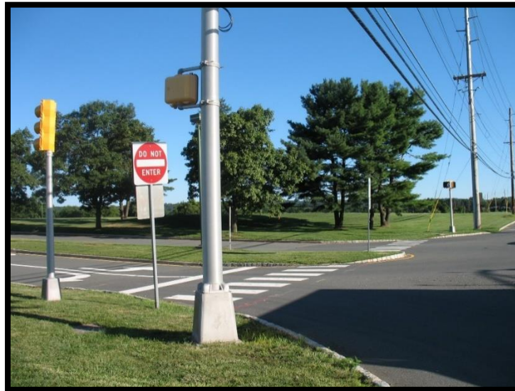
Lack of ADA compliant pedestrian accommodations
