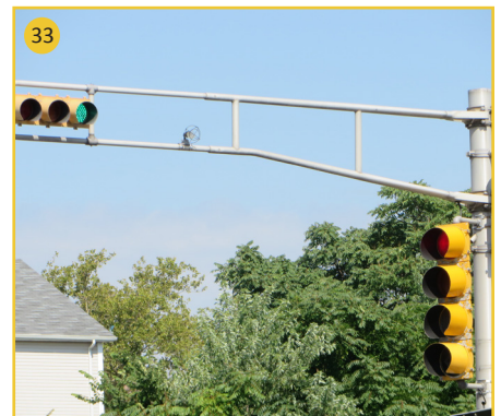
The 8-inch signal heads are not as visible as the 12-inch heads
