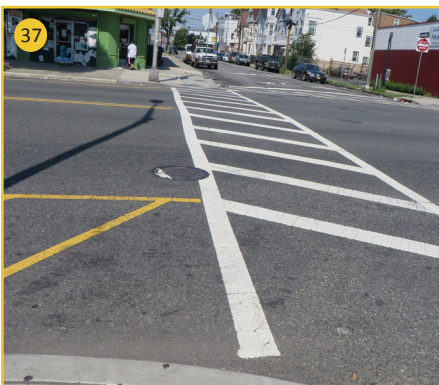
Very wide crosswalk is often unsafe to cross
