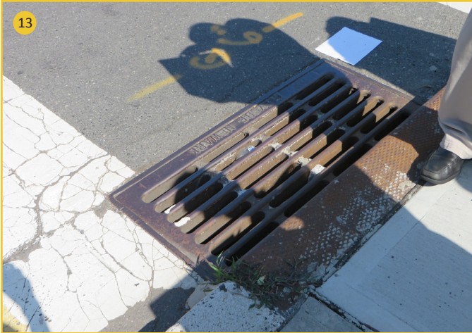
Inlet grates are not bicyclesafe
