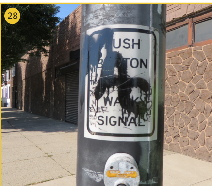
Pedestrian push buttons are not operational
