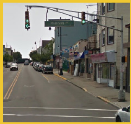
There are no southbound merge signs or pavement markings on south leg.
