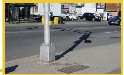
There are no northbound merge signs or pavement markings on the north leg.
