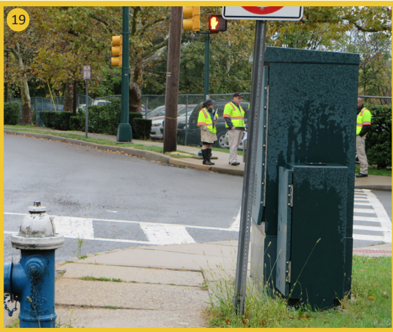
Figure 20 – Controller box limits visibility
