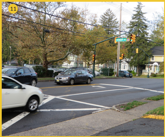
Figure 22 – Stop bar located back from intersection
