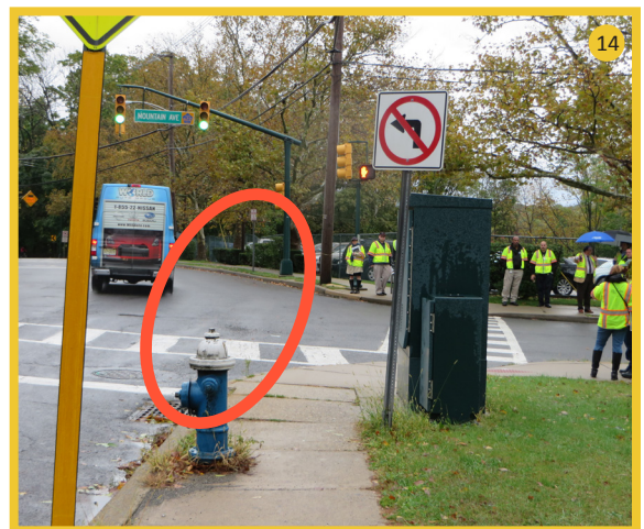
Figure 27 – The southern curb line isn't aligned
