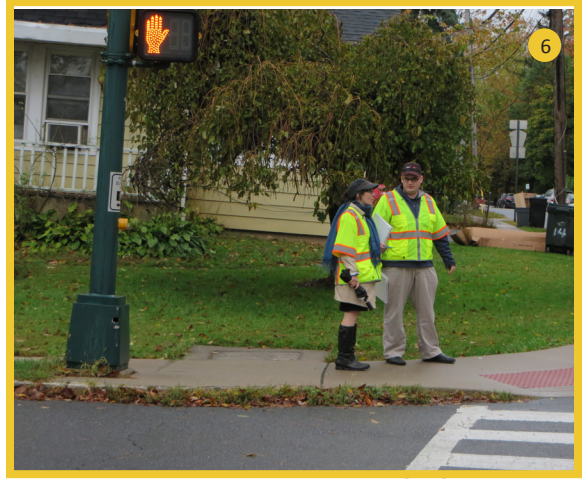
Figure 21 – Pedestrian push button far from landing
