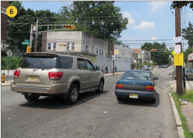
Unclear lane delineation and extra width of the single lane in each direction along 18th Avenue leads motorists to treat it as two lanes.
