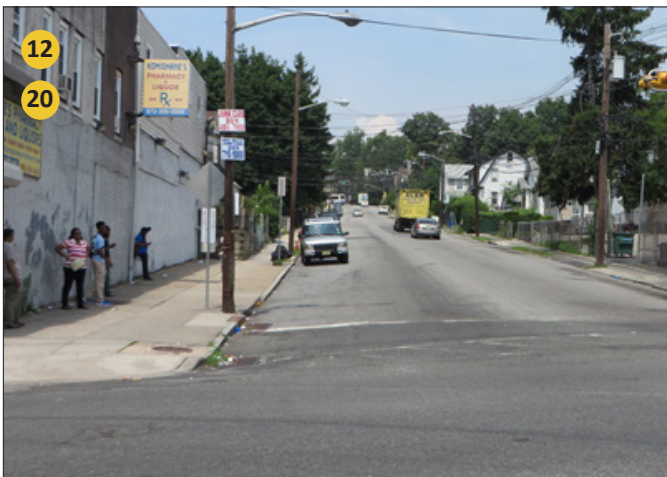
Faded crosswalks and centerline; No bus shelter or benches.
