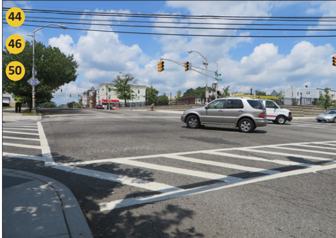
Vertical curve may limit motorist visibility; long crosswalks across Park Avenue; negative offset on Park Avenue.
