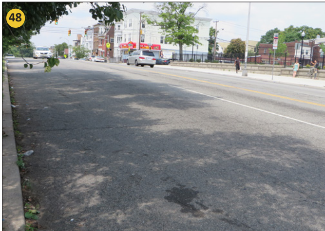
Wide outer lanes (~18') may contribute to increased speeds, especially as the curbside parking spaces seem underutilized; lack of bus shelters or benches.
