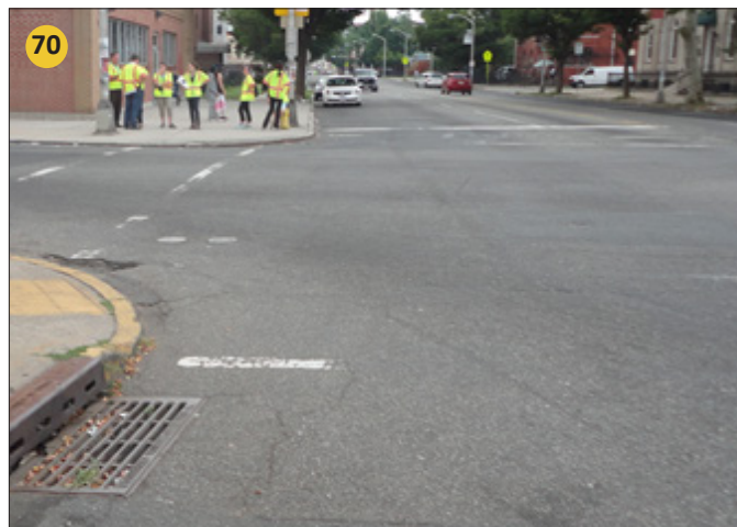
Faded pavement markings; crosswalks not high visibility.
