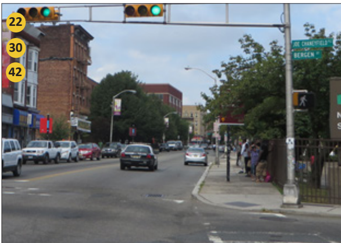
Wide receiving and bus lane is a confusing merge point for motorists. Lack of bus shelters or benches, despite high ridership.
