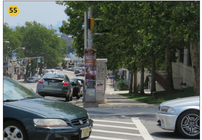
Foliage blocks pedestrian signal head.
