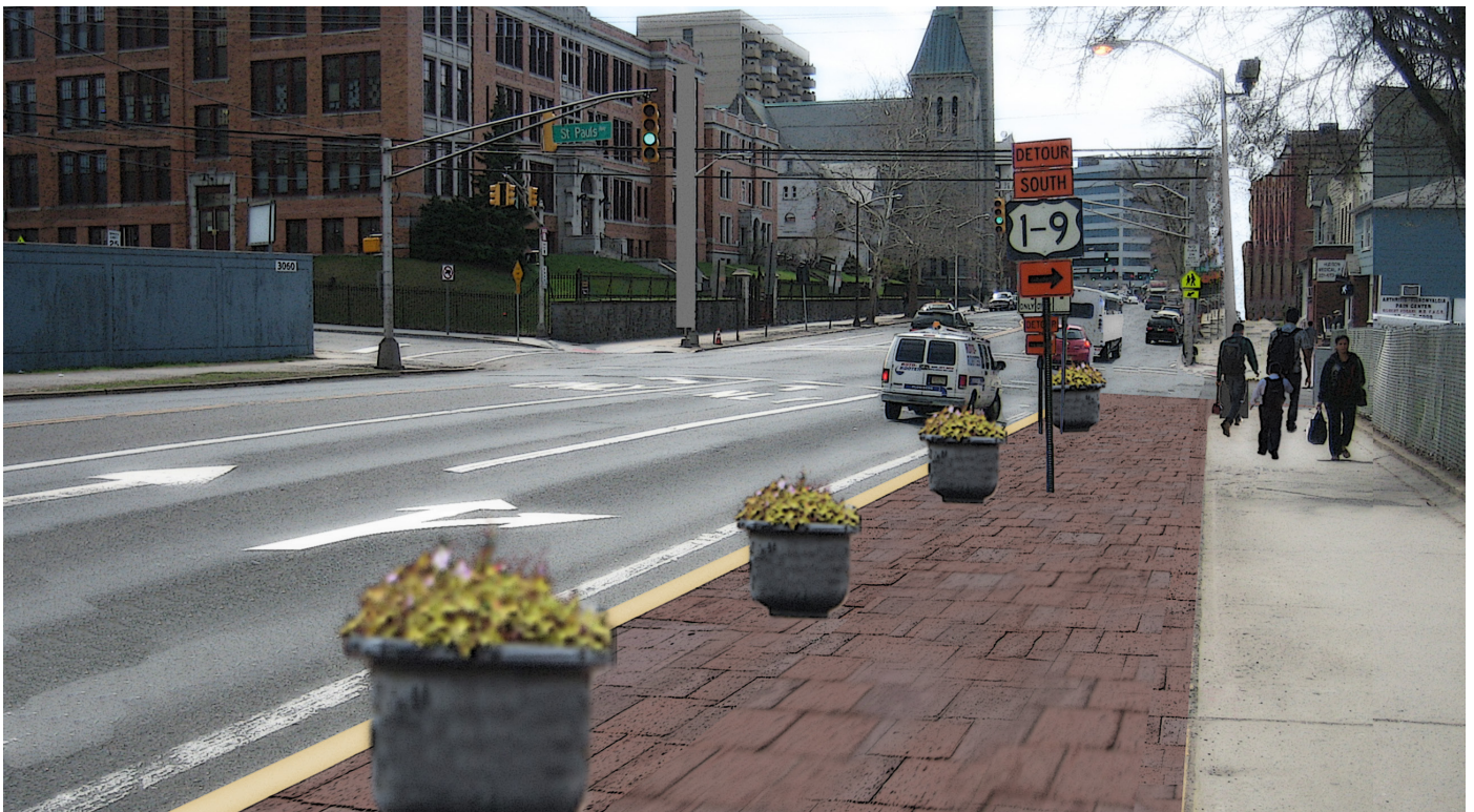
Figure 25 – St. Paul's Avenue & Kennedy Boulevard looking southbound, with right-turn lane removed, sidewalk extended, added green space.
