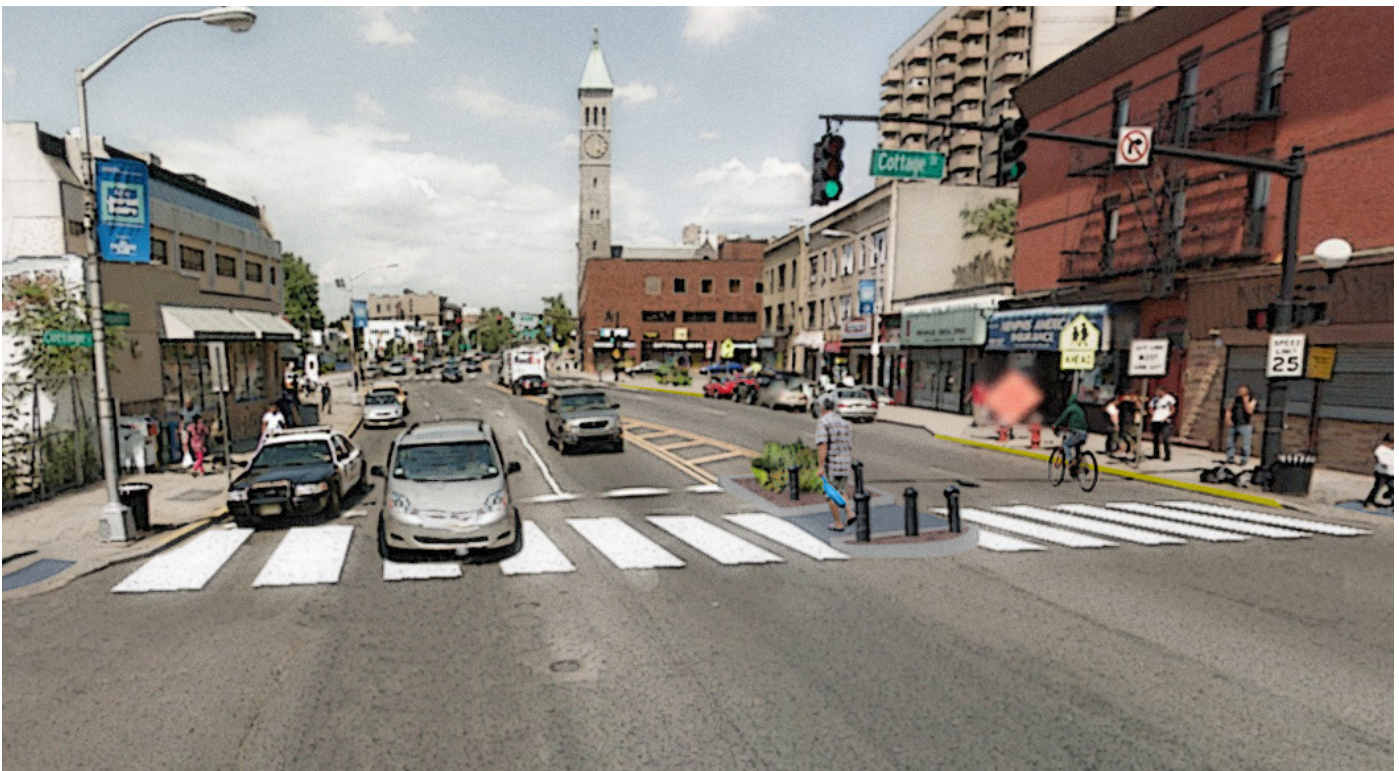
Figure 23 – Cottage Avenue & Kennedy Boulevard looking northbound, with refuge island, truncated domes, repainted crosswalk, removed merge sign, and curb extension along north leg (photo-simulated improvements).
