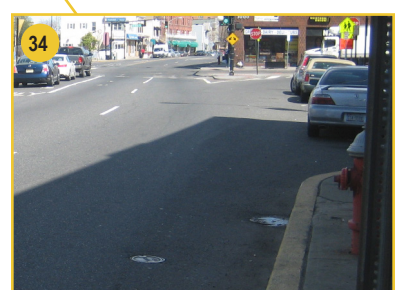
Right and through lanes on northbound approach are not clearly marked. Nor is there a parking delineation.
