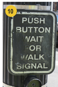
Some pedestrian push buttons were not properly oriented and appeared to be underutilized by pedestrians crossing the street.
