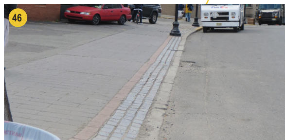
46 Prolonged depressed curb exposes pedestrians to vehicles turning into the adjacent parking lot.
