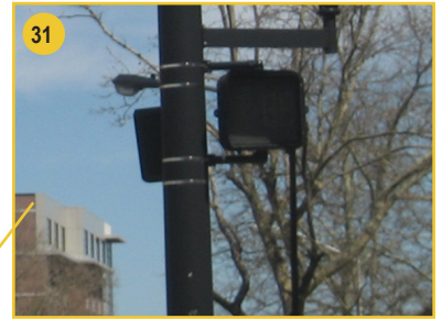
Broken pedestrian signal head.
