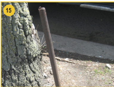
Abandoned pole near tree.
