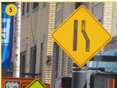
5 Misplaced merge sign.
