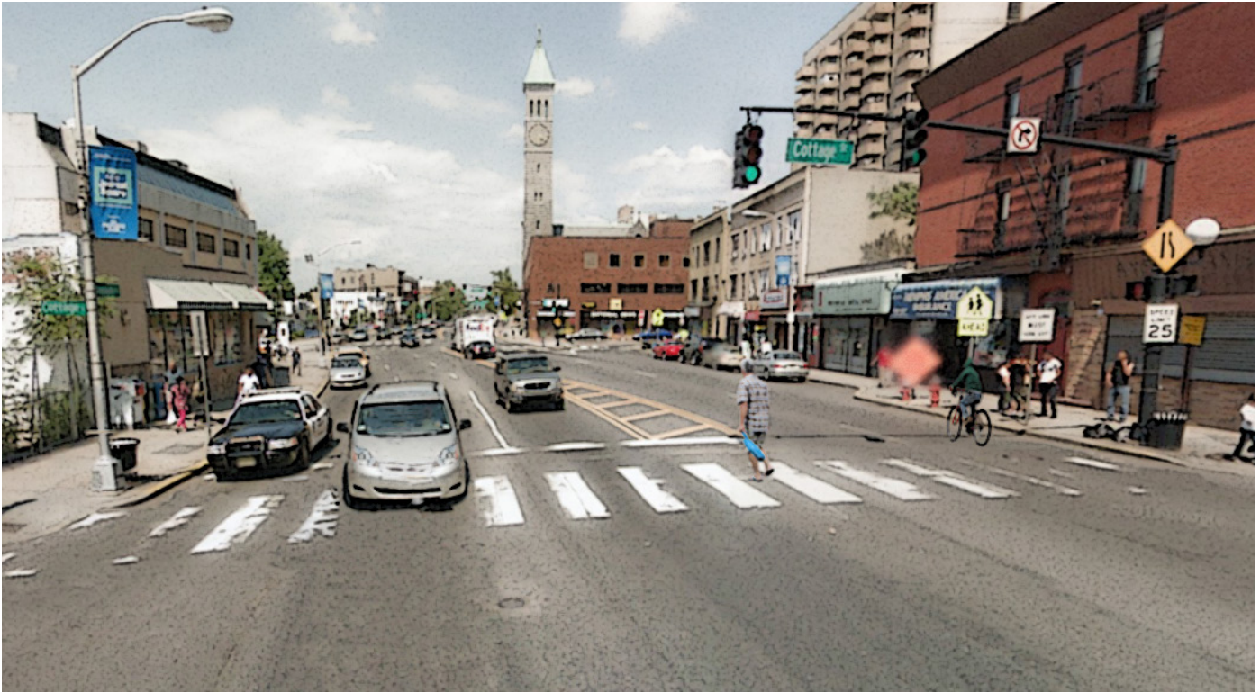
Figure 22 – Cottage Avenue & Kennedy Boulevard looking northbound (current).
