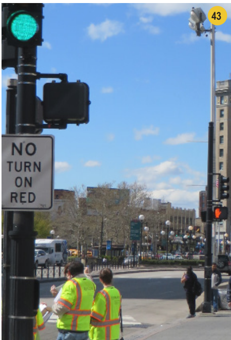
Some pedestrian push buttons were not properly oriented and appeared to be underutilized by pedestrians crossing the street.
