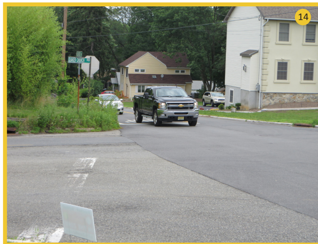
Figure 38 – Poor visibility on northwest corner
