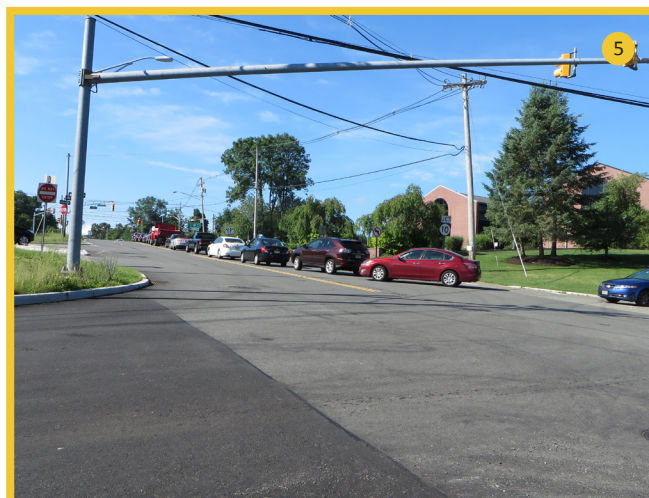
Figure 41 – Traffic backs up from the Rt. 10 intersection
