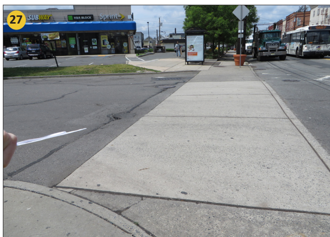
Insufficient differentiation between the wide driveway entrance (with long turning radii) and the sidewalks
