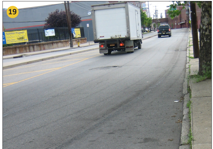
Wide lanes tend to have higher speeds and provide space for more aggressive passing maneuvers.
