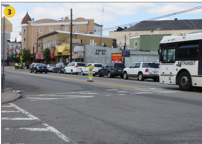
Crosswalk and other pavement markings are fading and need repainting.
