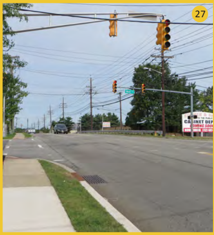
Reduced visibility due to vertical curve
