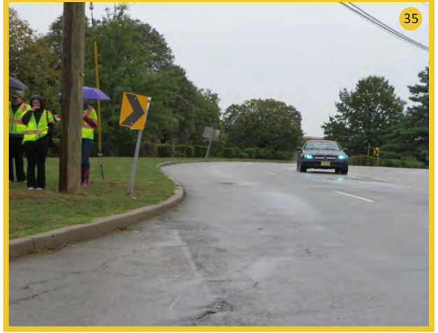
Chevrons and other indicators of the curves are lacking
