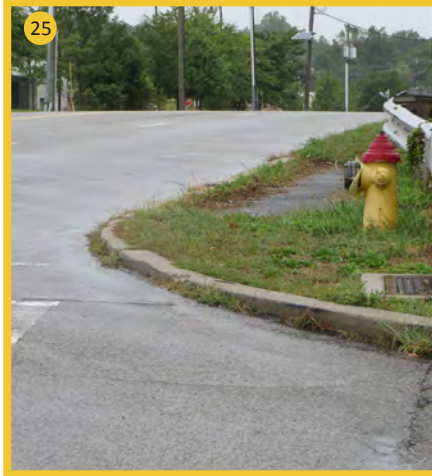
No ADA facilities on the north side of Allwood Road
