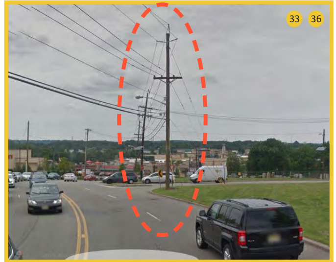
Utility pole has been struck numerous times as cars come around the curve
