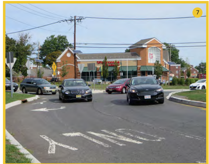
Poor lane delineation
