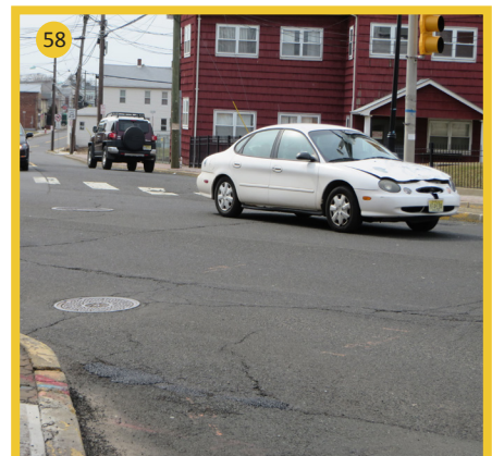
Conflict between left-turning vehicles and through vehicles
