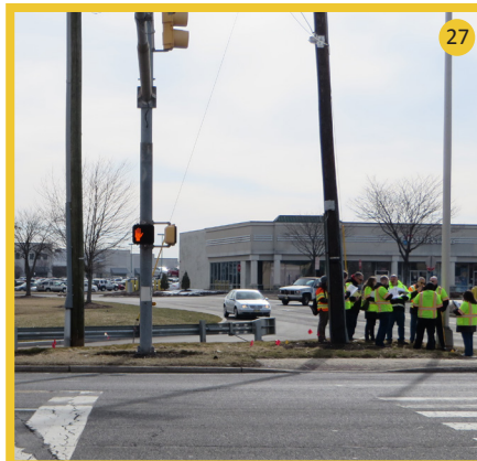
There is no sidewalk connecting to the crosswalk
