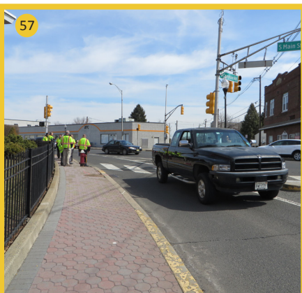
The large radius encourages making the turn at high speed
