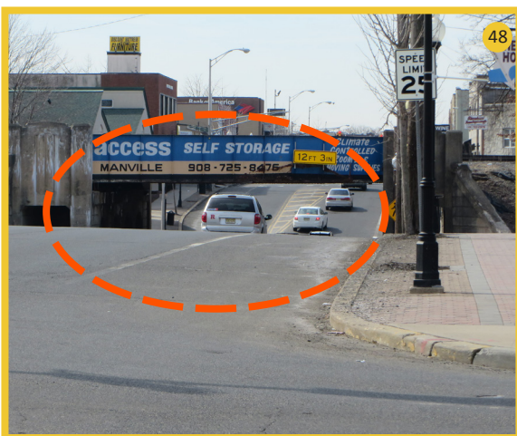
Vertical curves limit sight distance
