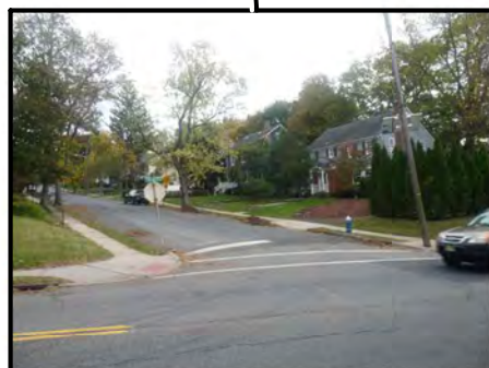
Lack of crosswalks and pedestrian signage
