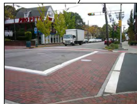
Outdated traffic lights and non-standard crosswalks
