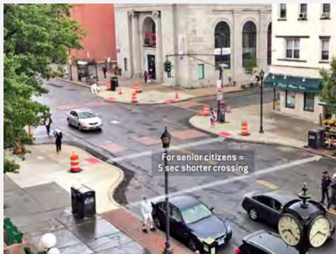
Curb Extensions Hoboken City, Hudson County
