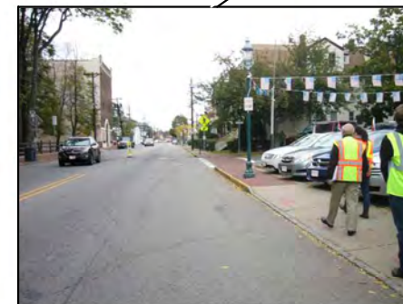
Observed speeding along corridor; non-standard pedestrian crosswalks
