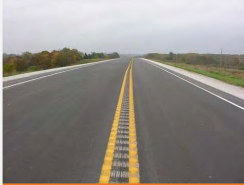
Longitudinal Rumble Stripes/ Center Line Rumble Stripes (CLRS)
