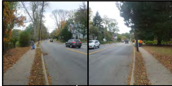
Limited sight distance due to roadside vegetation, road geometry (Left: NB, Right: SB)
