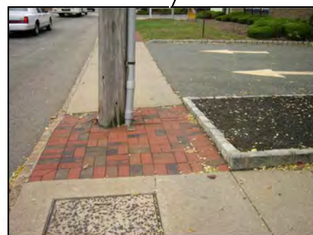
Sidewalk is narrow, obstructed, and uneven
