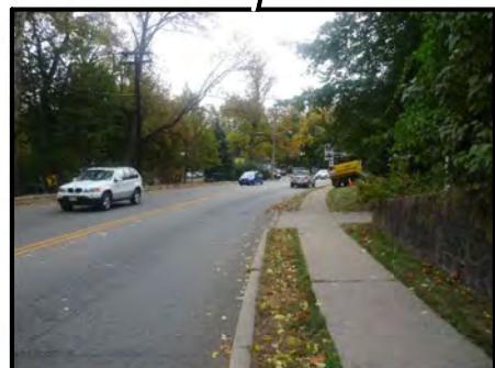
Limited sight distance for signalized intersection at Oakland Rd
