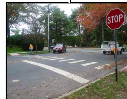
Stop bar far from intersection
