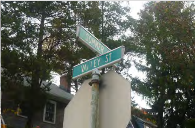
Worn signing and non-breakaway posts
