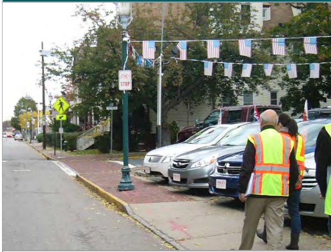
Poor pavement conditions and obstructed sidewalks
