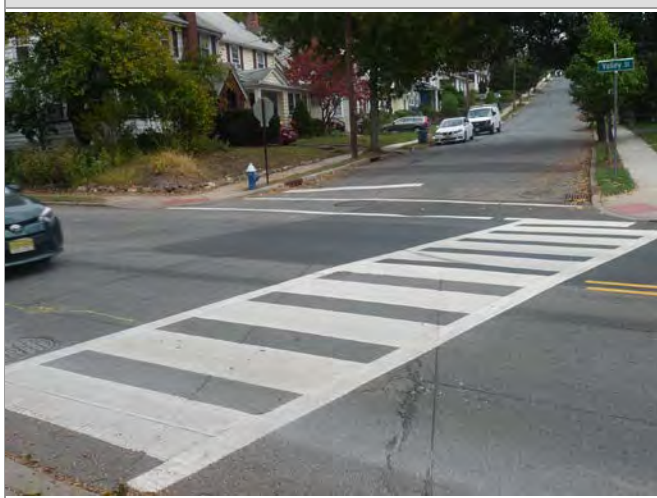
Marked crosswalk with no warning signs
