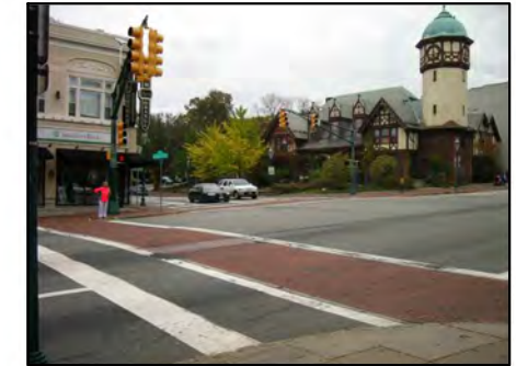
Wide pedestrian crossings, Poor sight distances, Ped heads are blocked by street signs
