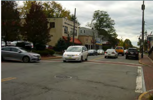
Limited sight distance and visibility at 2nd Street
