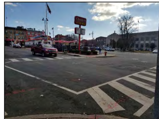
The wide roadway and lane configuration creates many conflict points for pedestrians and vehicles.
