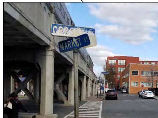
Many signs in the area are faded, poorly placed, or outdated.
