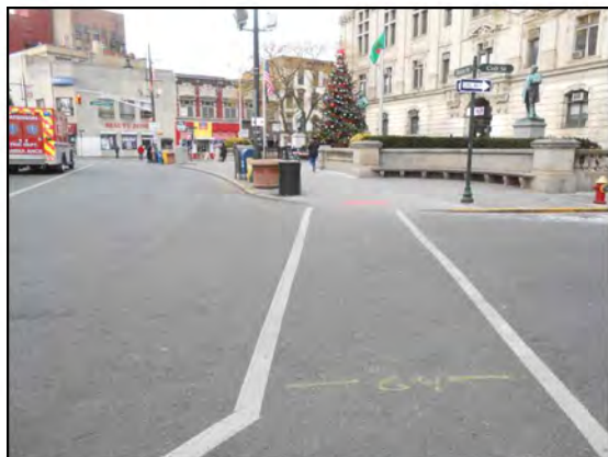
Wide outside lane with no delineation for the adjacent bus stop. Faded yellow no parking curb.
