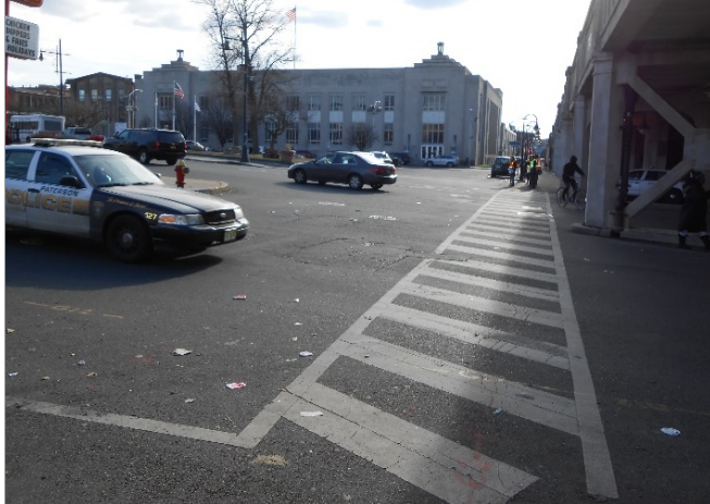
The Crosby Pl, Park Ave, and Market St is extremely wide and lacks traffic control devices
