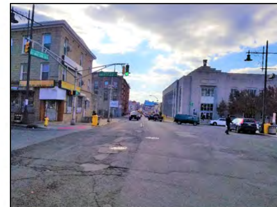
The pavement is in poor condition and the lanes are poorly delineated.
