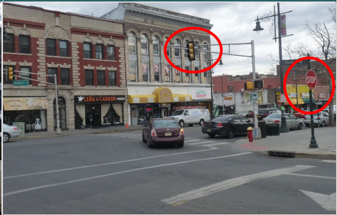
Signal heads at Clark St are not operational; conflicting traffic control may cause confusion
