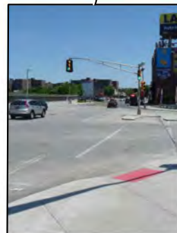
Worn striping on structure
