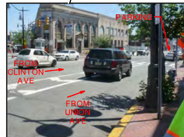
Lack of available merge distance on Clinton Ave southbound
