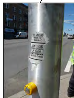
Push button stickers worn/peeled away
