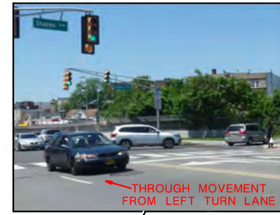
Lane use change between closely spaced intersections confusing to motorists
