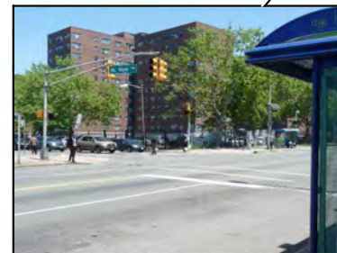
Major pedestrian crossing and bus stop lack high visibility crosswalks
