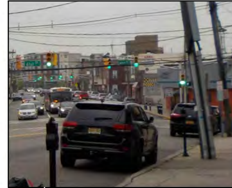
Overhead utilities obscure some signal heads
