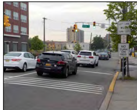
No advanced curve or signalhead warning Signs are not mounted at proper height
