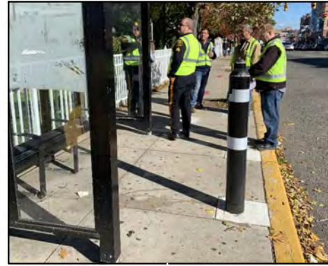
Bollards encumber pedestrian path around bus shelter
