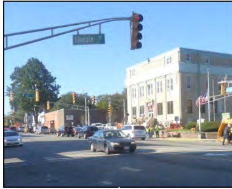
Lack of "pull-through" signal indications for JFK northbound may confuse motorist
