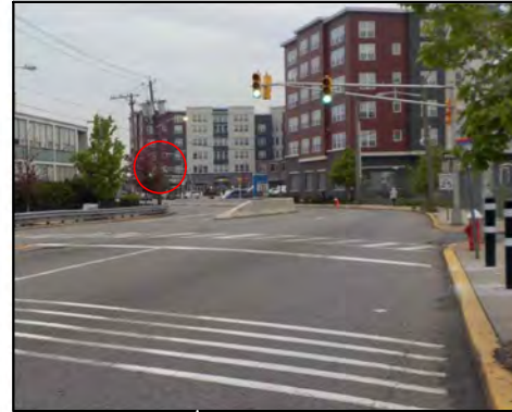
Signal heads for adjacent intersection are obscured by vegetation and curve
