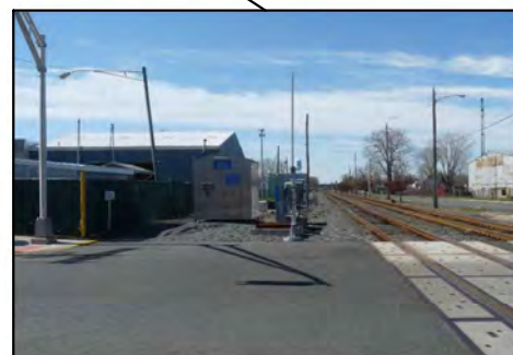
Unclear pedestrian path (lack of sidewalk)
