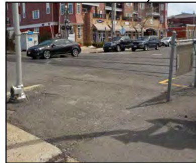
Pedestrian path not well defined near rail crossing/across tracks
