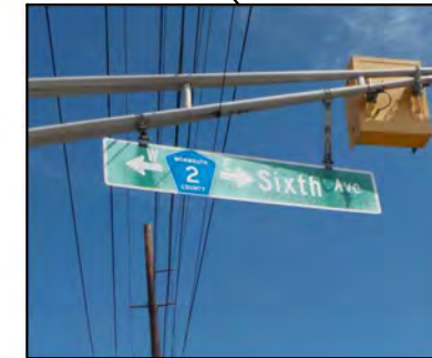
Faded mast arm signs
