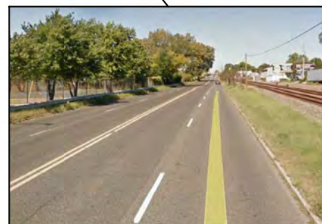
No shoulders or lighting
