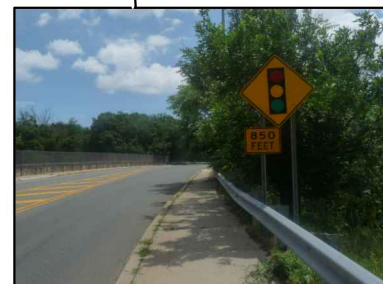
Limited visibility EB of Highland Parkway intersection (over GSP)
