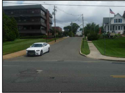
No ADA curb ramps, DWS, crosswalk, stop sign or striping
