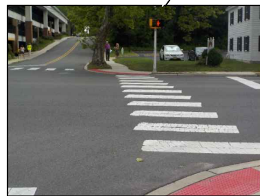
Use of DWS around entire curb radi may be confusing to vision impaired
