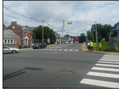
Vehicles make wide left turns at higher speeds; no ADA curb ramps
