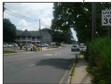
Lack of/narrow shoulders, utility poles within pedestrian path, and limited sidewalk width increases driver and pedestrian discomfort
