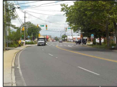
Vegetation, geometry and inadequate lighting may obscure pedestrians in crosswalks
