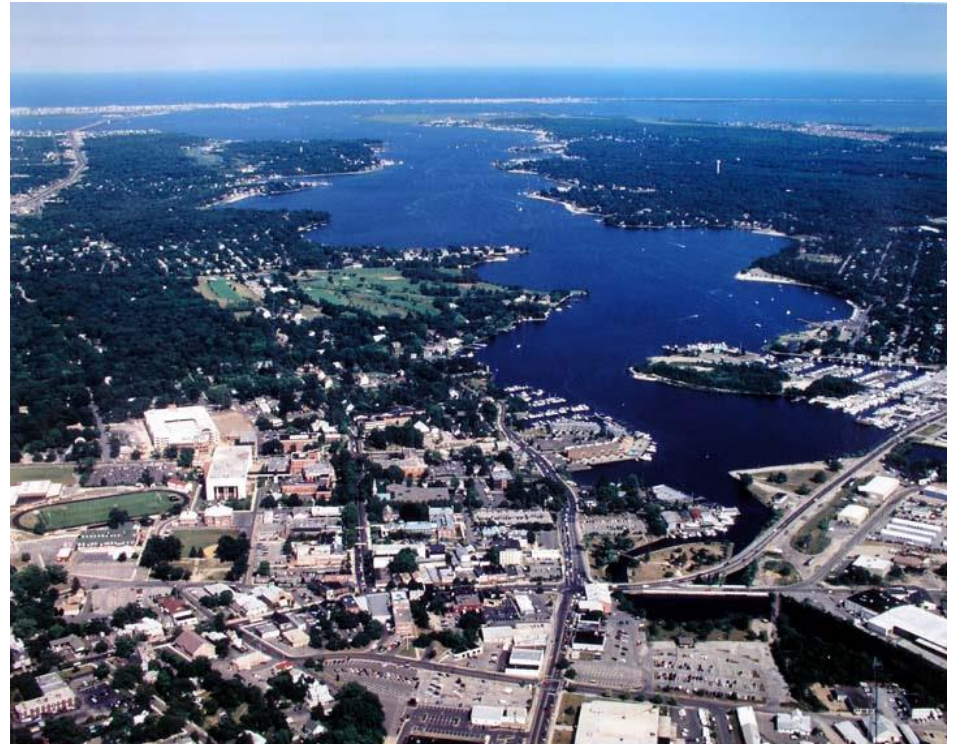
Figure 2: Aerial view of Downtown Toms River facing east towards Barnegat Bay.
