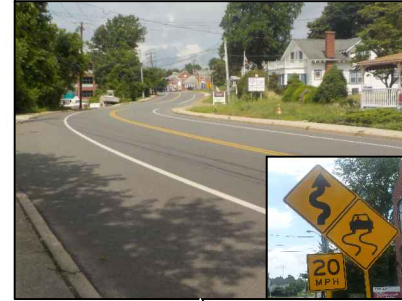
Sidewalk abutting curb is narrow (inset: advanced curve warning signs west of Hooper Ave)
