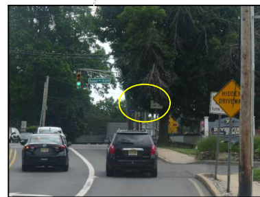
Signs obscured by vegetation and close spacing
