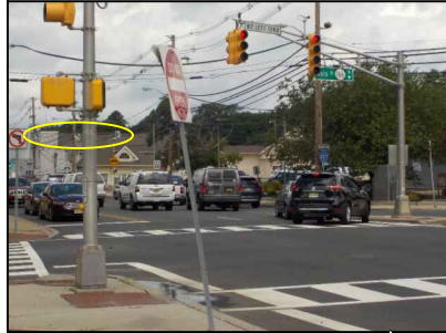
Lane configuration at Irons St results in de-facto weaving section where SB channelized right enters
