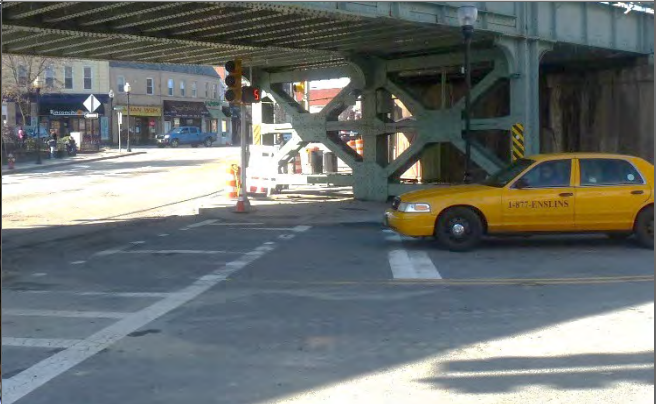
10. Crosswalks need restriping
