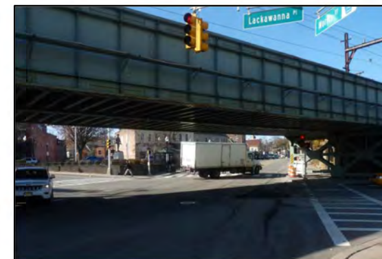
Train bridge obstructs intersection visibility
