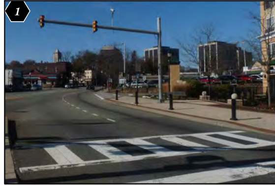
Lane use approaching next intersection not clear; curb ramp lacks detectable warning surface
