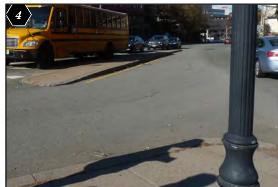
Median and channelized island shapes create narrow turning area
