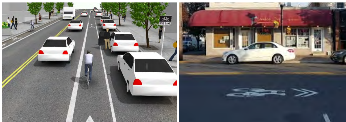
Figure 12 – Bicycle Facility Examples
