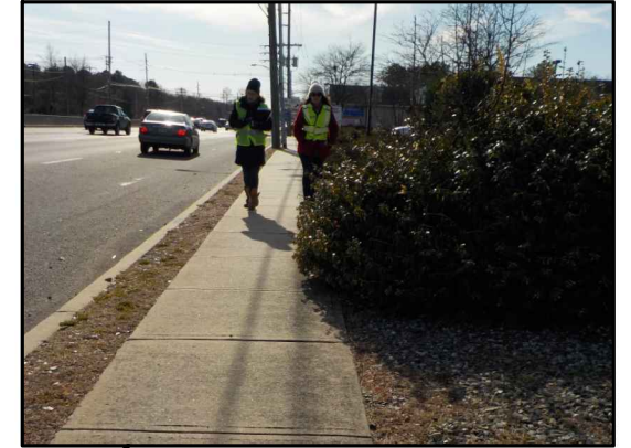
Overgrown shrub needs trimming; reduces usable width of sidewalk
