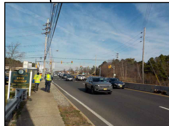
Wide shoulder and bus stop area can be restriped to indicate bus stop
