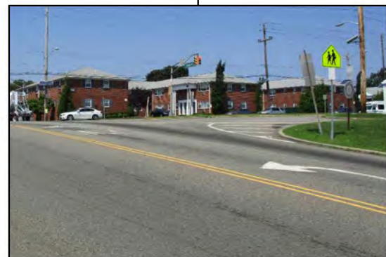
Large corner radius at cemetery entrance increases pedestrian crossing distance and right turn speeds
