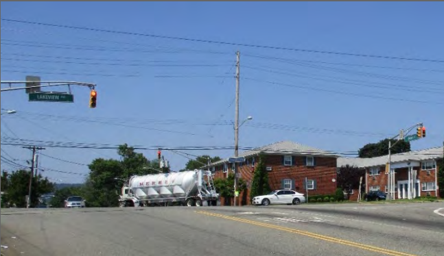
9. Signal heads can be upgraded to 12" with backplates for better visibility
