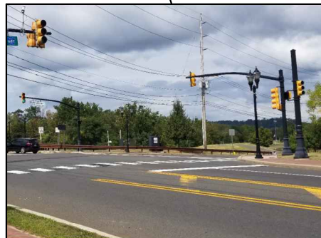
Worn gore striping due to EB alignment through intersection
