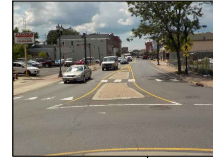
Low roundabout splitter islands do not provide sufficient definition or refuge and lack detectable warning surfaces
