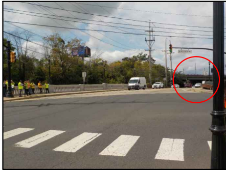
Visibility of signal traveling WB may be obstructed by structure
