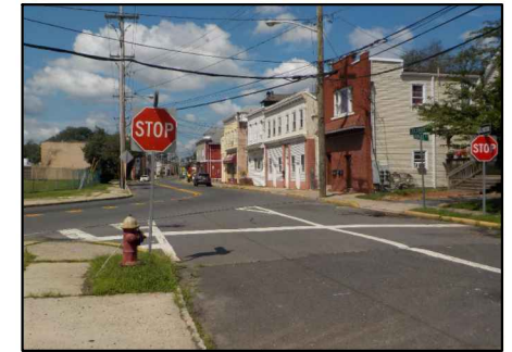
Intersection lacks ADA ramps; driveway within intersection
