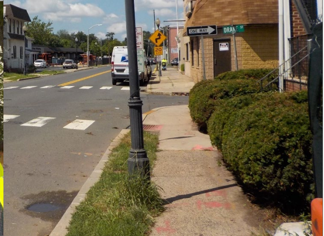
8. Shrubbery needs trimming
