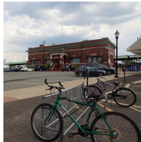
Bicycle Parking at Bound Brook Train Station
