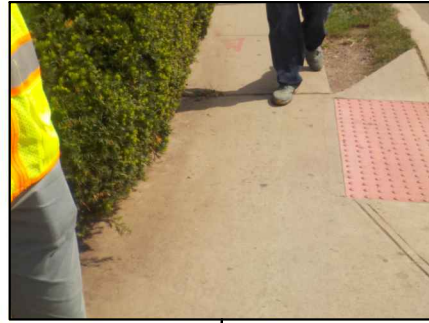
Landscaping overgrown onto sidewalk, reducing walking path
