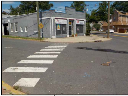
Sight distance limited by building; wide intersection with long pedestrian crossing
