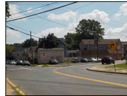
Roadway horizontal alignment limits sight distance along CR 533 and at Talmage Ave
