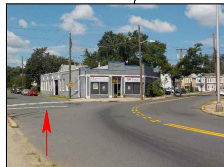
Roadway horizontal alignment limits sight distance along CR 533 and at W Main St; stop bar in front of crosswalk
