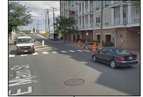
Long pedestrian crossing at Meridia parking deck difficult to see; wide driveway lacks clear definition
