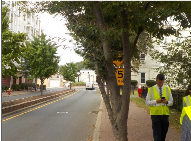
7. Visibility of roundabout sign impeded by trees
