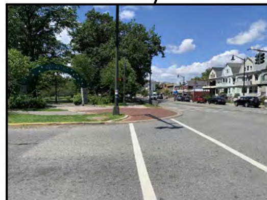
Crosswalk leads directly into driveway for the park
