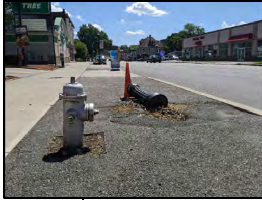
Damaged fixtures create tripping hazards for pedestrians
