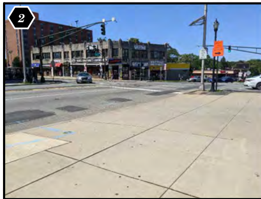
Access management; driveway located immediately adjacent to the intersection
