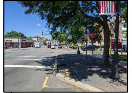
Trees block visibility of signs and signals
