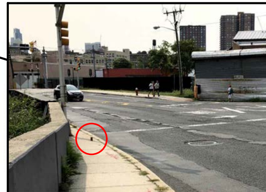
Narrow sidewalk with tripping hazard
