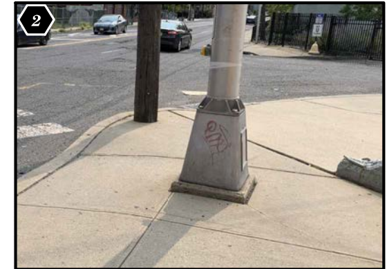
Objects in sidewalk create obstacles with little passing room
