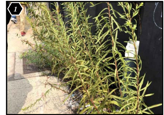
Overgrown vegetation restricts use of full sidewalk width
