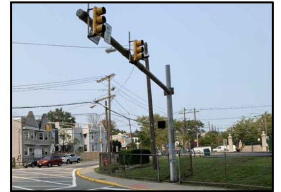
No street name signs and 8-in signal heads
