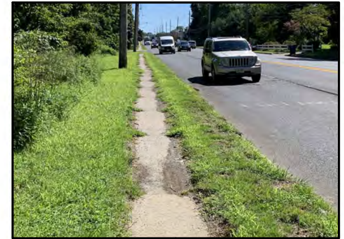
Vegetation overgrowth limits sidewalk No shoulders along corridor
