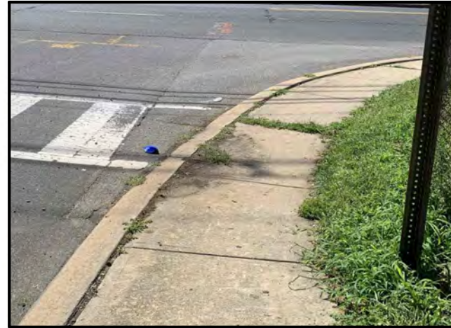
Various sidewalk widths and conditions
