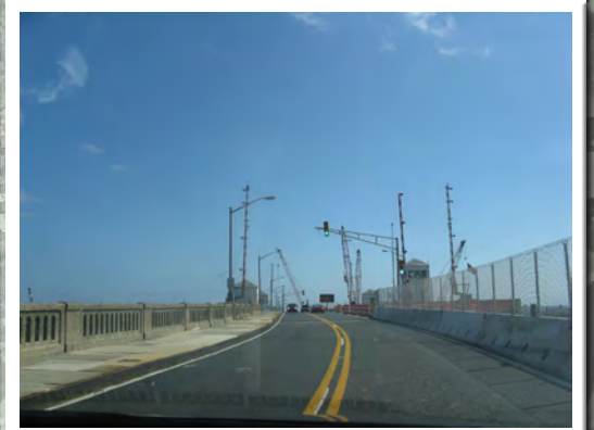
Highlands Bridge Primary Gateway that provides link South from Highlands Borough to Sea Bright Borough linking Bayshore to the Coastal Region. Historic design elements could be augmented with decorative lighting and artist treatment on bridge walls.
