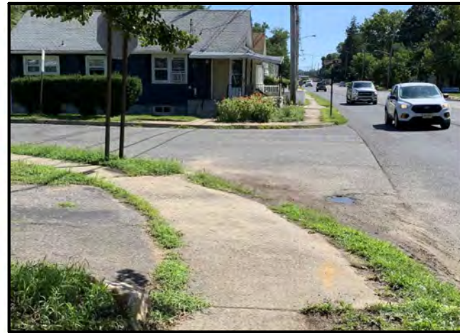
Unclear use as driveway or sidewalk Not ADA compliant
