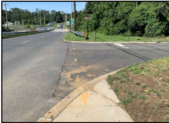
Sidewalk does not continue west of Munson Pl
