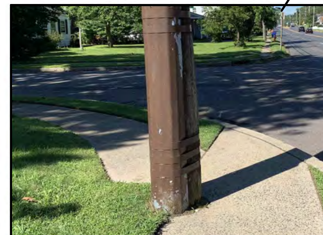
Curb ramps not ADA compliant
