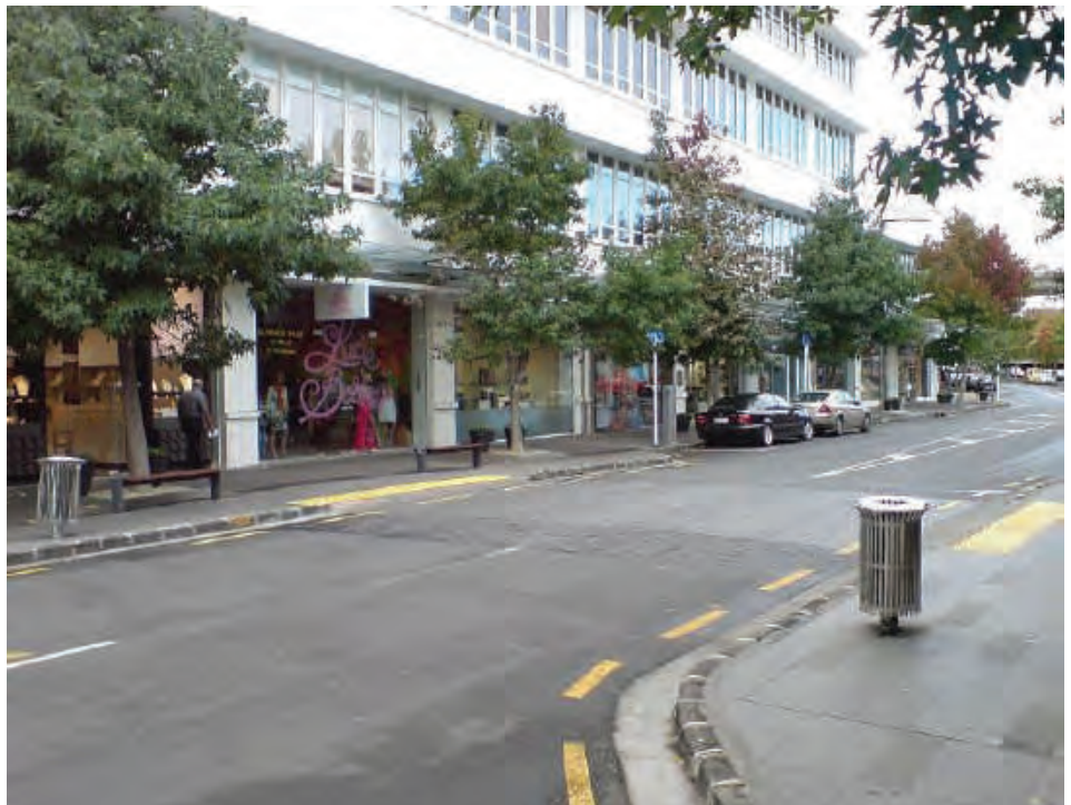
A speed table creates an at grade mid-block street crossing while also slowing vehicle speeds. Source: NACTO.org
