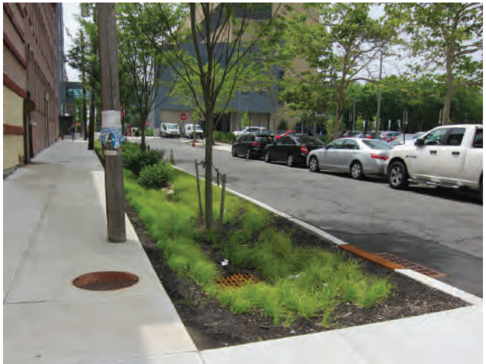
Green stormwater infrastructure along Summit Street on NJIT's campus collects and filters rainwater, cleaning the water and slowing its entrance into the City's sewer system.
