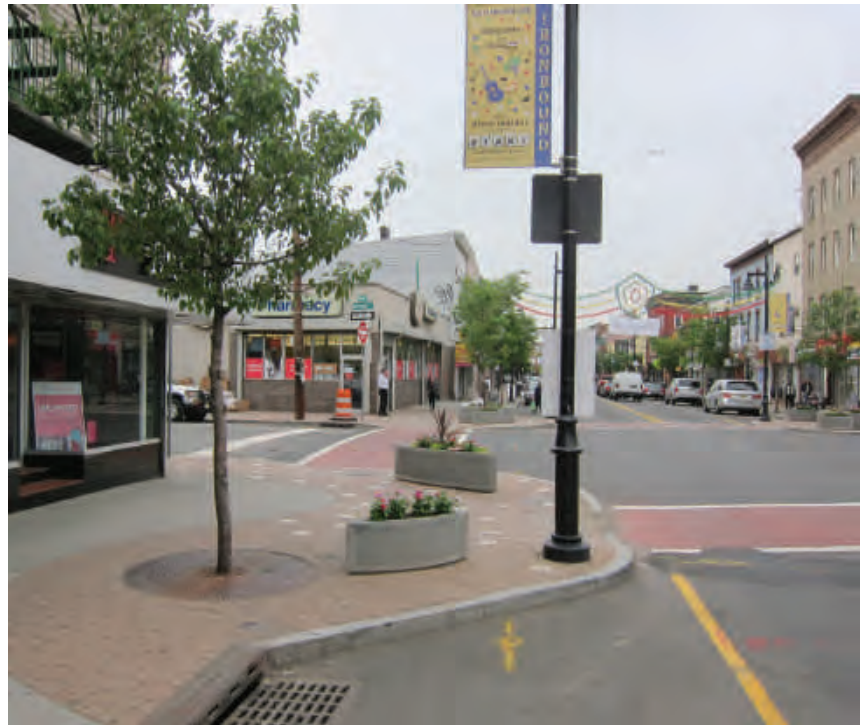
Ferry Street - Corner bump outs shorten the crossing distance and improve pedestrian visibility.
