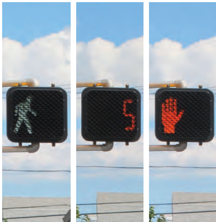
Wilson Avenue - A countdown signal displays the time remaining to cross the intersection.
