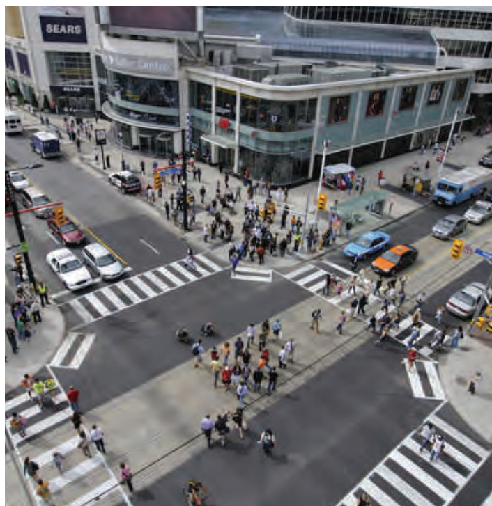
An exclusive pedestrian phase stops all directions of traffic and allows all pedestrian to cross simultaneously, including diagonally. Source: buryinc.com
