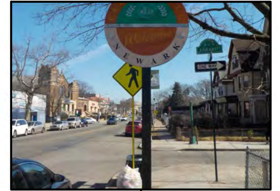
Pedestrian crossing not clearly marked with striping; sign obscured
