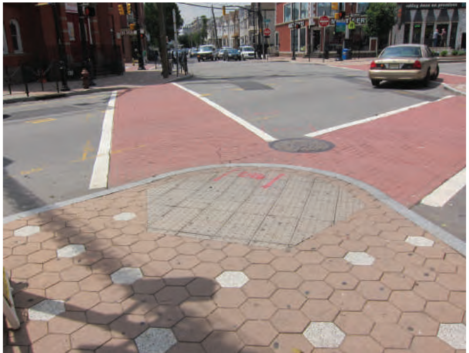
Ferry Street - Curb ramps on Ferry Street ensure ADA compliance, providing access between the sidewalk and the street for people who use wheelchairs or with pushing strollers.
