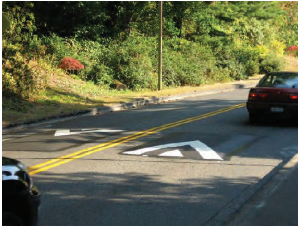
A speed cushion allows large vehicles such as buses and firetrucks to pass the speed hump unaffected. Source: NACTO.org
