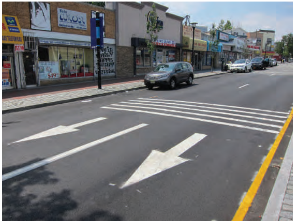
Bloomfield Avenue - Rumble strips alert drivers to an upcoming signal and reinforce slower speeds.
