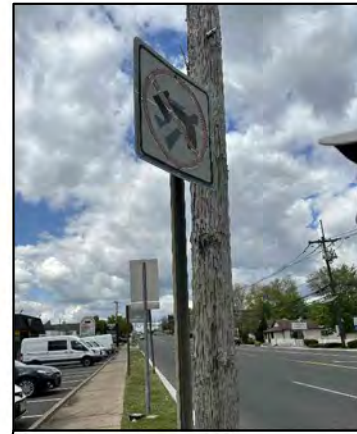
Faded no left turn sign
