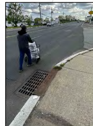
Missing ADA curb ramps; No crosswalk and stop bar markings; Large curb radius
