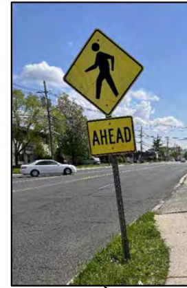
Faded pedestrian ahead sign with low vertical clearance
