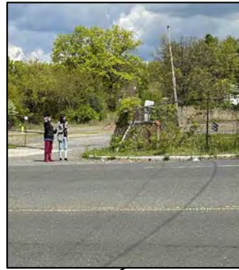
Missing sidewalk, curb ramps and crosswalk
