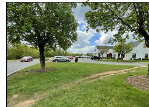
Worn travelpath across Wells Fargo building
