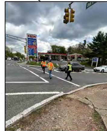
Non compliant ADA curb ramps; Each crosswalk approach does not have a separate curb ramp
