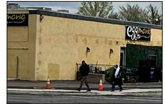
No physical barrier or vertical curb between sidewalk and driveway
