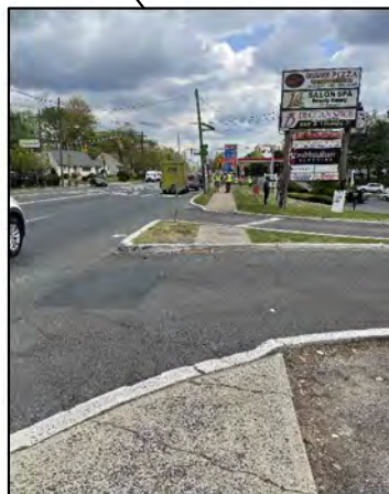
No marked crosswalk; Missing ADA curb ramps
