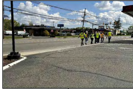
No offset between sidewalk and roadway
