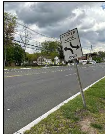
Center turn lane sign tilted
