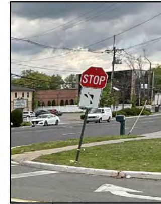
Faded no left turn sign; Stop sign tilted
