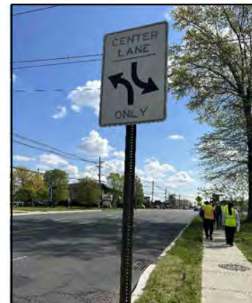
Faded two-way center turn lane sign
