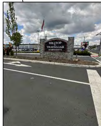
Establishment signs and vegetation obstructing sight lines; Incorrect thru arrow pavement marking
