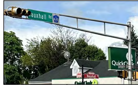
Outdated traffic signal equipment
