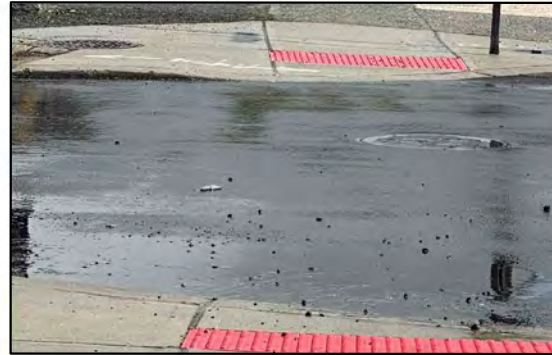
No marked crosswalk; Missing stop bar marking
