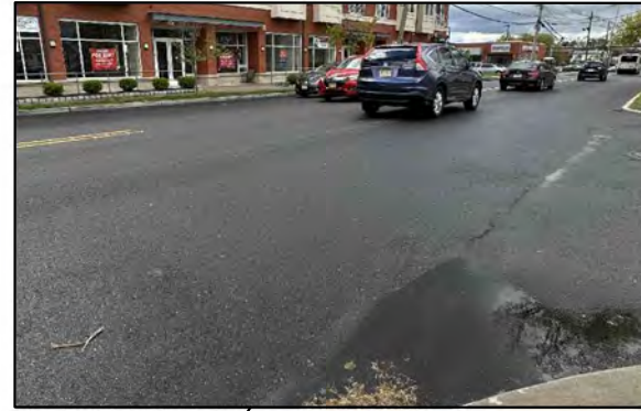
No marked crosswalk across Stuyvesant Avenue despite bus stop presence
