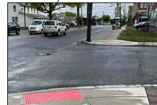
No marked crosswalk; Missing stop bar marking
