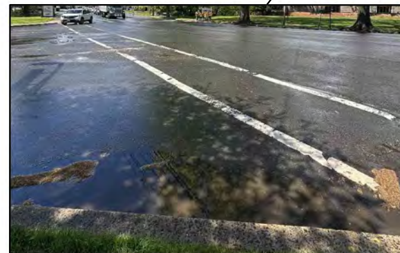
Long pedestrian crossing and faded crosswalk; Large curb radii; No pedestrian signal equipment
