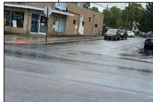
No marked crosswalk; Missing stop bar marking
