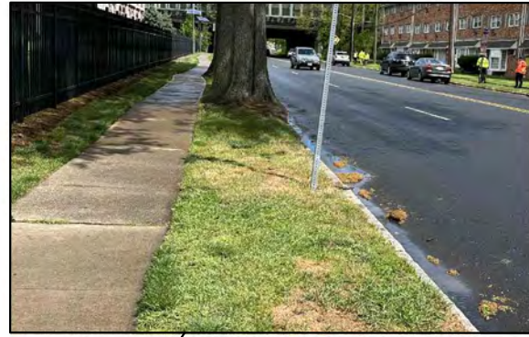
Tree protruding beyond curb
