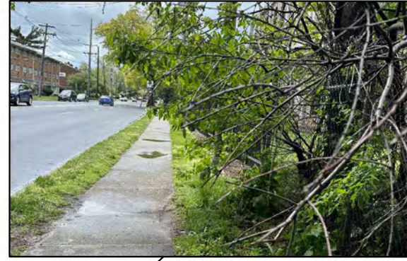
Vegetation obstructing sidewalk
