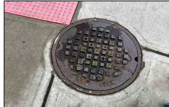
Manhole in ADA curb ramp area
