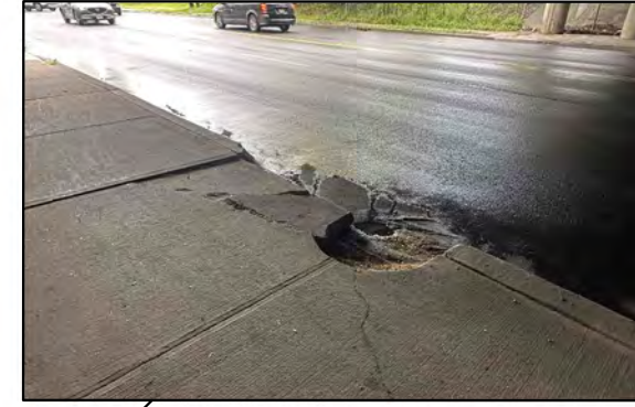
Sidewalk curb cut out for manhole maintenance
