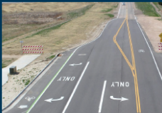
Left- and right-turn lanes on a two-lane road. Source: City of Greeley, CO
