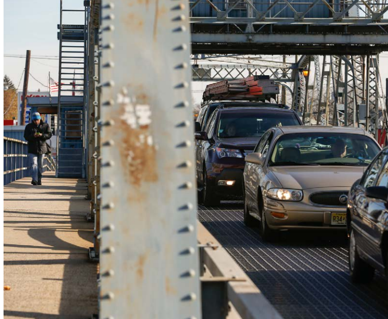
Kingsland Avenue Bridge, Bergen/Essex Counties
